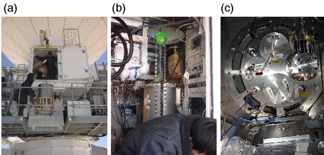
**Fig. 7.** (a) A photograph of carrying the receiver system into the receiver cabin. (b) A photograph before installation of the receiver system. (c) A photograph after installation. Bottoms of three cartridges and the cryocooler are seen. The warm IF amplifiers and bias electronics are not mounted.
