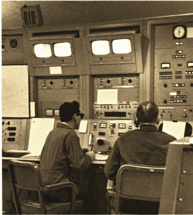
Part of the control complex for the Rohr-built 210-foot diameter deep space tracking antenna.
