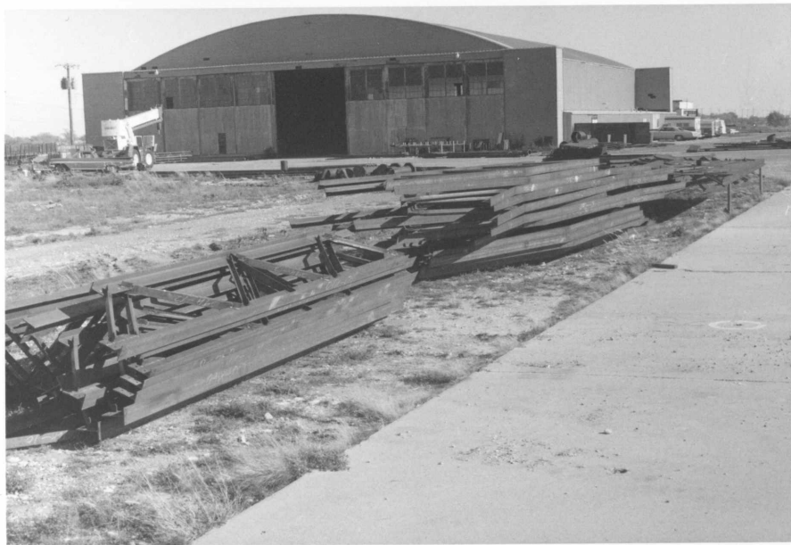
(p11-5) 11/20/74 - View of E-Systems antenna fabrication plant at Hobbs, New Mexico, belonging to Structures, Inc. Note completed antenna reflector truss parts stored in foreground.
