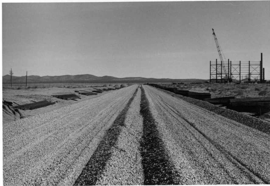
(p11-1) 11/15/74 - View of Wye to Northeast showing railroad ballast. Note rail spread at left, ties to right, Antenna Assembly Building in background.
