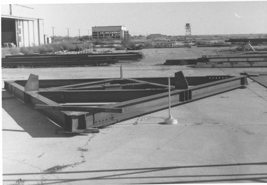
(p11-6) 11/20/74) - View of completed triangular base for Antenna No. 1.
