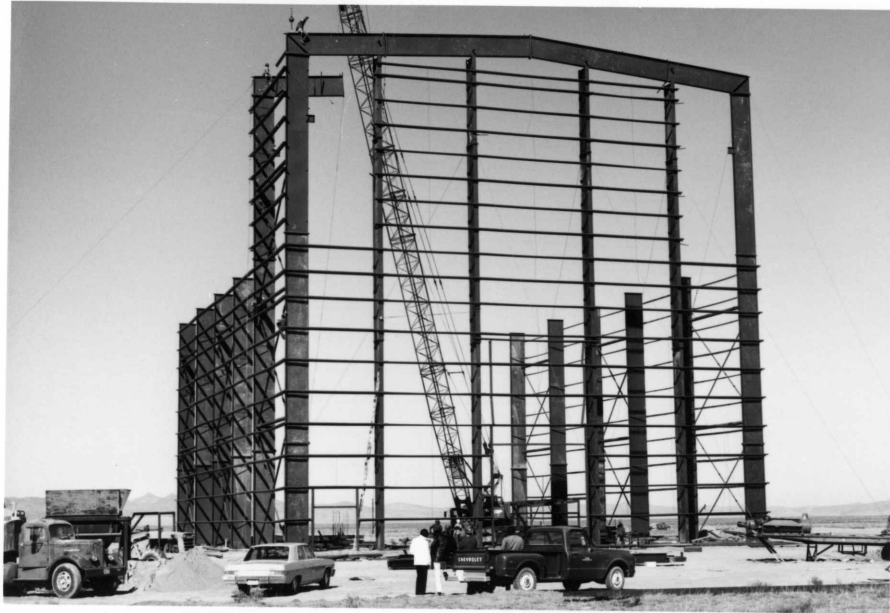
(p11-3) 11/20/74 - Steel erection at Antenna Assembly Building.
