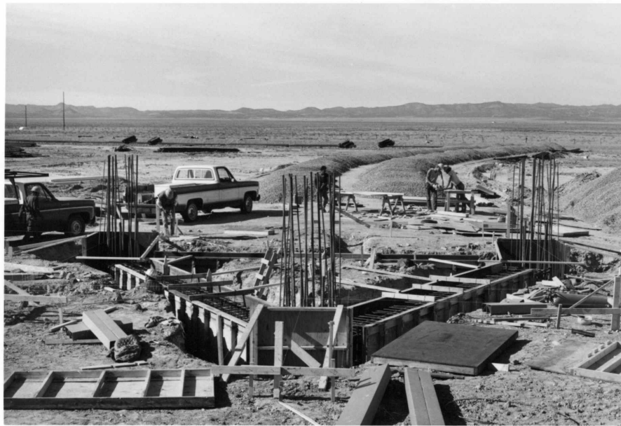
(p11-2) 11/15/74 - View of maintenance area antenna station form work and reinforcing steel. Note ballast spread in background.
