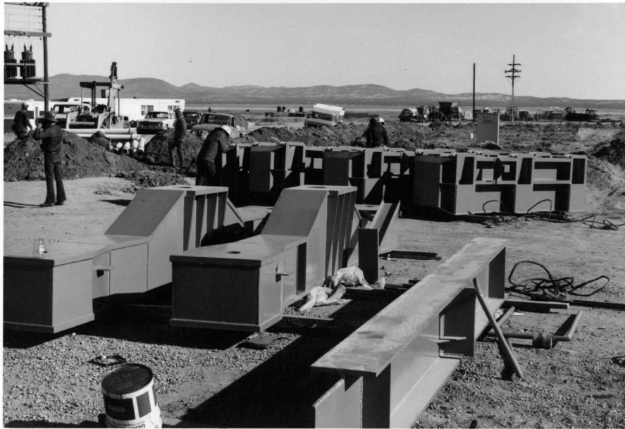
(pl-75-5) Transporter weldments at Site awaiting assembly
