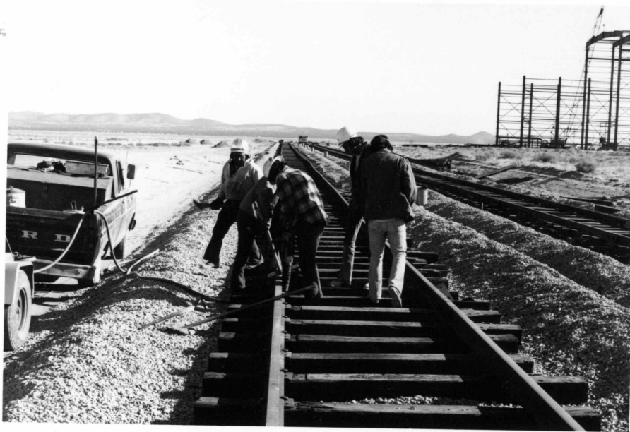
(p1-75-2) Spiking and preliminary alignment of the track
