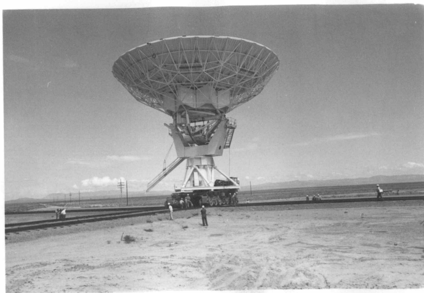
Antenna #1 on Transporter at Intersection with Main Tracks
