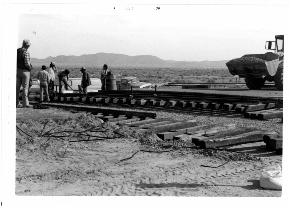
Placement of Rail Across U. S. Highway 60
