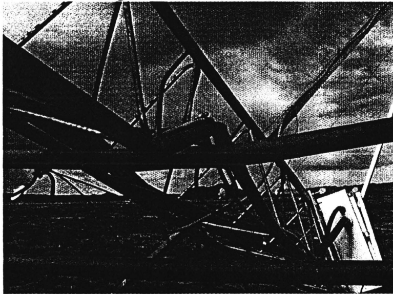
Mid-Tower Section After Tower Failure
