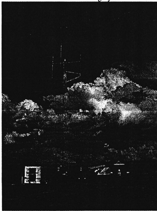
The EMS Tower next to the RFI Shelter
