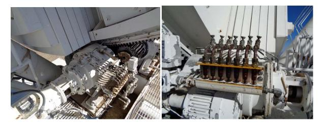
The duration of the maintenance visit the antenna structure was checked over for cracked welds, rusted members and overall condition. Bolts were spot checked for tightness with no loose bolts founds. Backup structure could use some touch up paint, but overall good condition. Welds and structure near elevation bearing showed no signs of cracking or fatigue. VTX room and external
