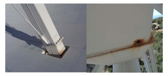
The dish surface was inspected and found to be free of major dents or holes. The paint is starting to fade in areas, as shown in pictures. Panel bolts were spot checked for tightness, all fasteners checked were still acceptable.
