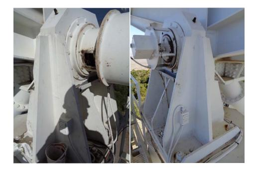
Both elevation platforms and catwalk were inspected. Overall in good condition. There are a few areas that can be touched up with paint, but structurally sound. Catwalk and pins, and all stairways on elevation platform appeared in good condition, other than could use paint as well. Jib-arm and joist looked in good condition, cable did not show excessive wear or frayed strands.
