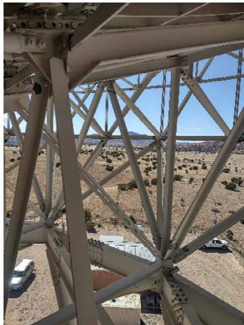
Figure 11: Dish Backup Structure Inspection
