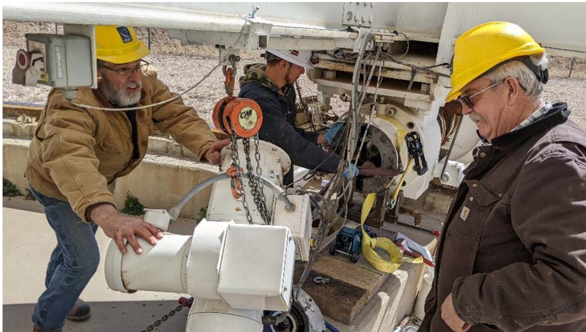
Figure 3: Rigging around motor assembly to pull off second motor housing.
