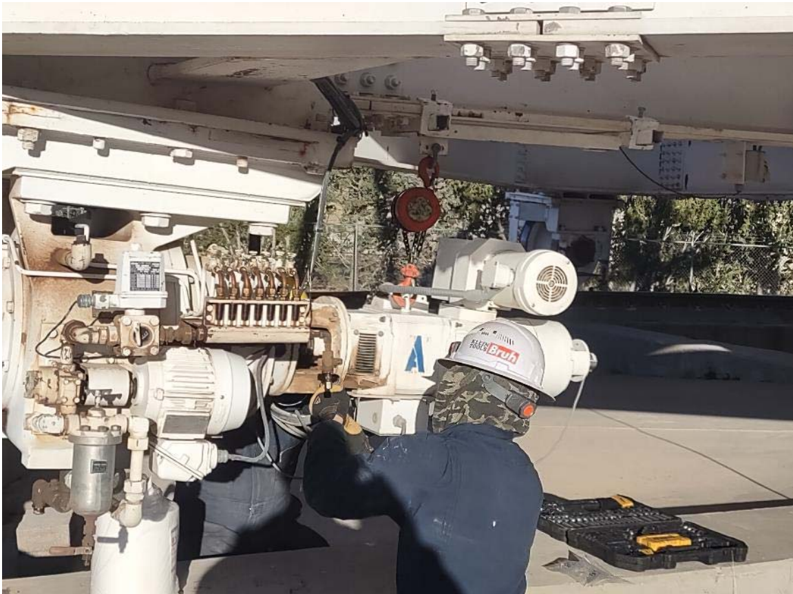
Figure 2: Pat and Carlos utilizing motor-brake assembly lifting device during removal
