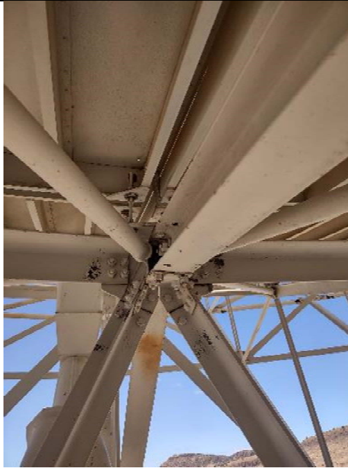
Figure 10: Dish Backup Structure Inspection
