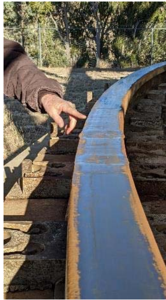
Figure 6: Rail Surface Deformation
