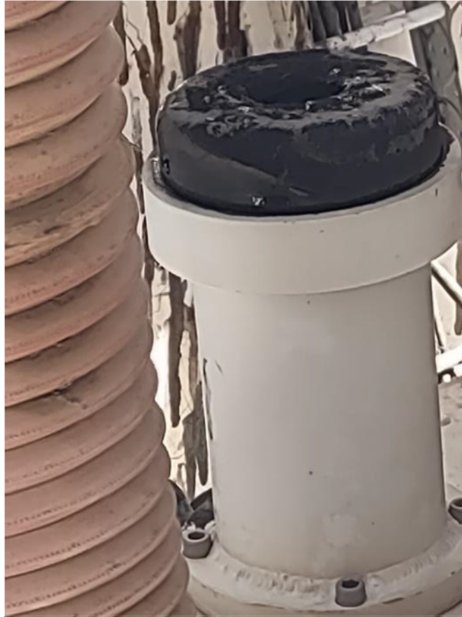
Figure 15: FRM Rubber Bumper Condition
