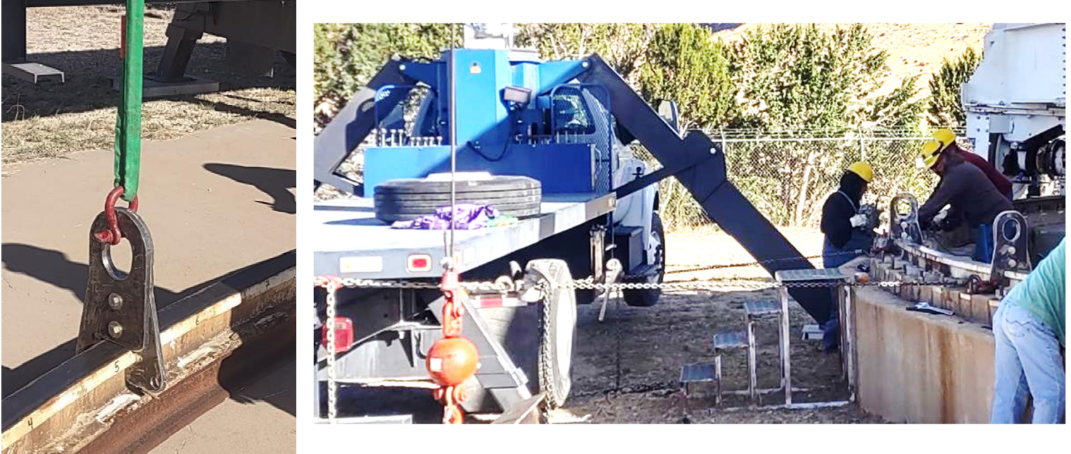
Figure 4: Rail Lifting Plates and Lever Puller Attachment
