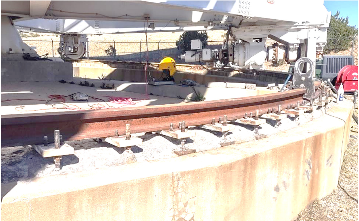
Figure 7: Old Grout Removed and Support Plates Exposed
