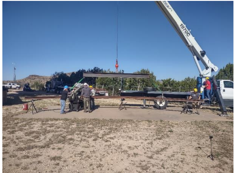
Figure 3: Saw cutting on concrete slab
