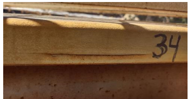
Figure 6: Delamination Crack Examples
