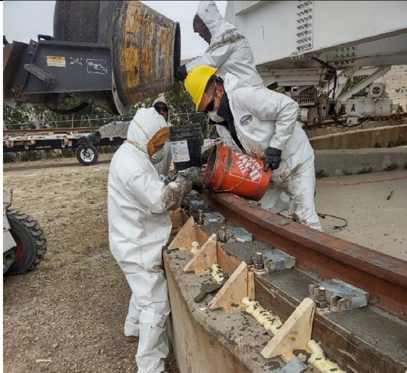
Figure 9: Pouring Epoxy Grout and Grout Forms
