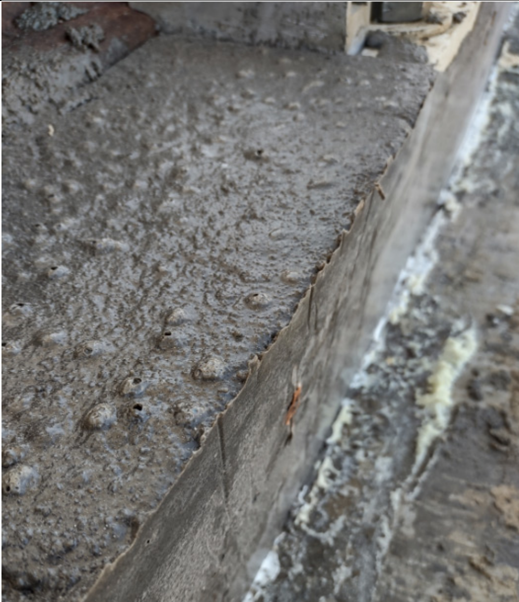
Figure 10: Cure Grout and Air Entrainment
