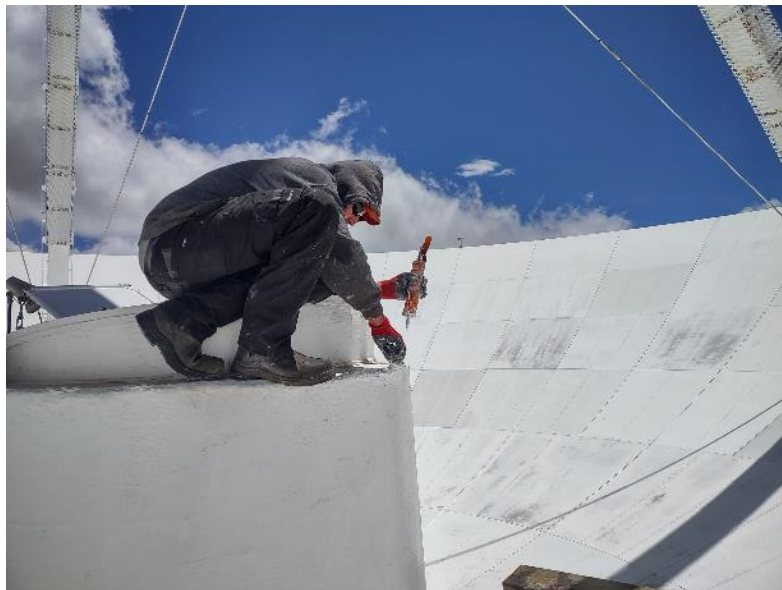
Figure 2: Repairing Ice Damaged Spots on Feed Housing
