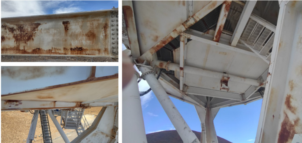
Figure 10: Corrosion Examples
