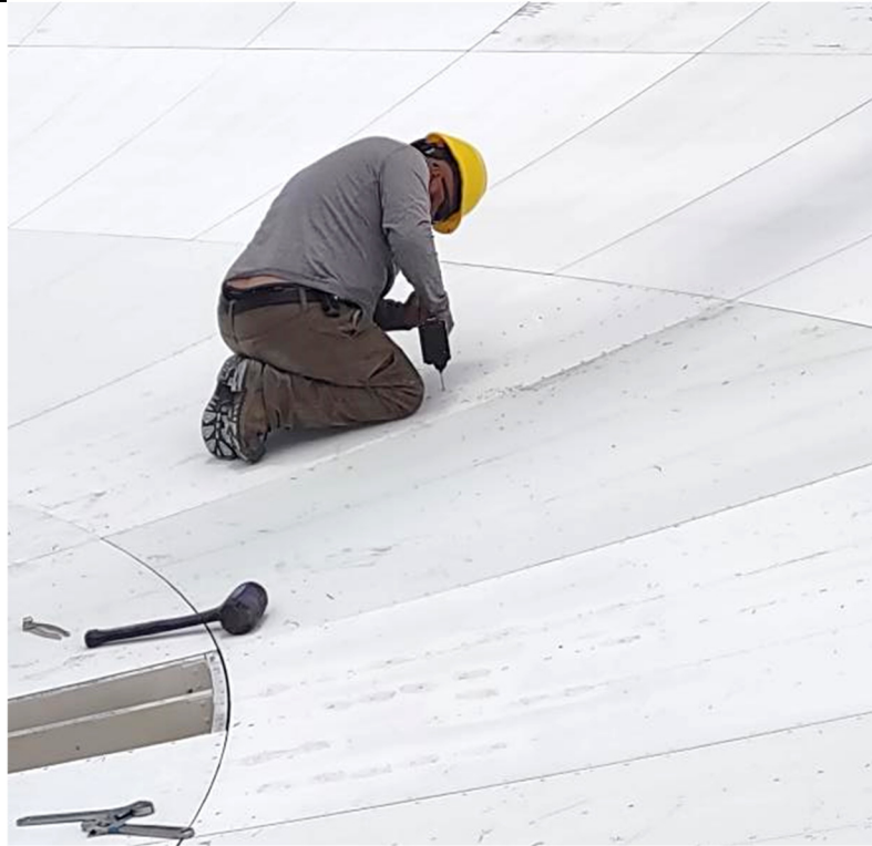
Figure 3: Drilling Out the Old Rivets
