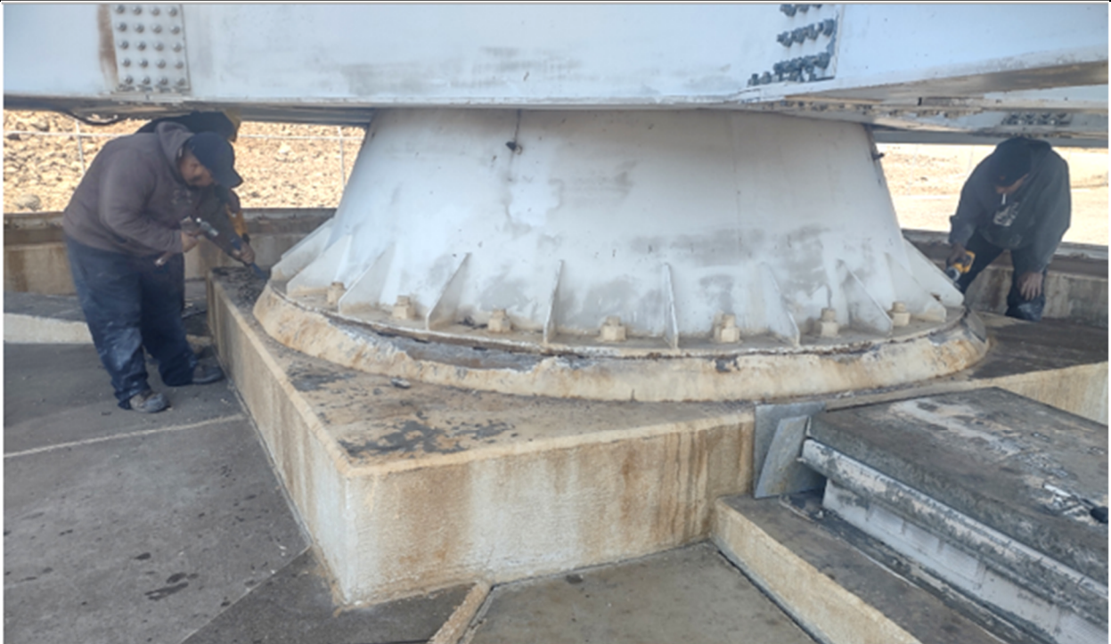
Figure 12: Mortar Fix Around Lower Pintle Bearing Structure
