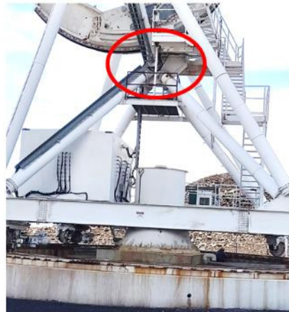
Figure 9: Boxed Area of Lower Structure
