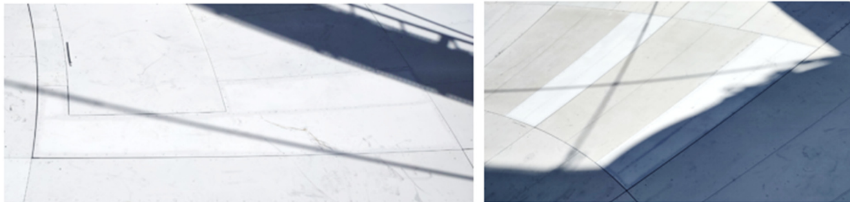
Figure 7: New Installed Panels
