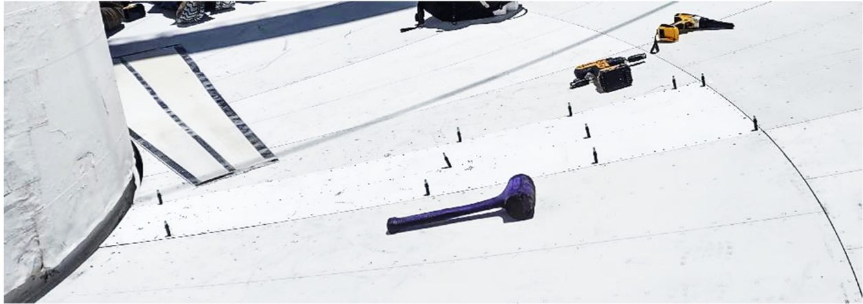
Figure 4: New Panel Retained with Clecos
