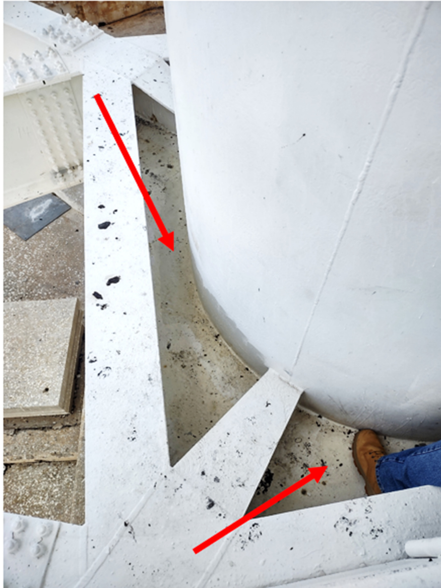
Figure 2: Upper Center Pintle Area Rust Repair
