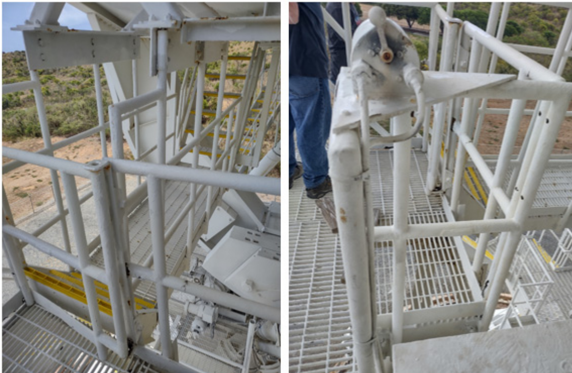
Figure 8: Swinging Catwalk Gate and Adjacent Hand Rail
