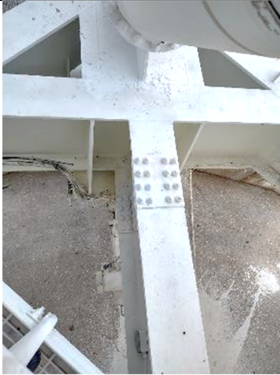
Figure 3: Example of Lower Structure Paint Maintenance
