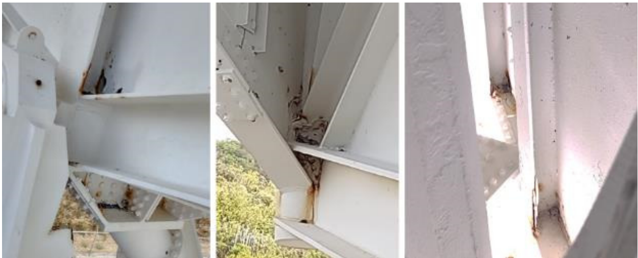
Figure 14: Structure Corners that need Closer Inspection
