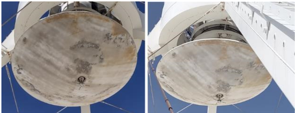
Figure 16: Condition of the Sub-Reflector
