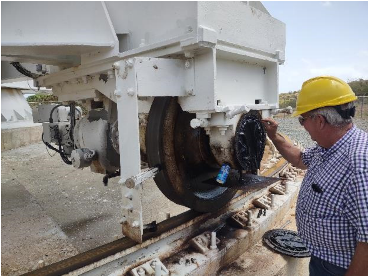
Figure 22: Az 2 Outer Wheel Bearing Inspection
