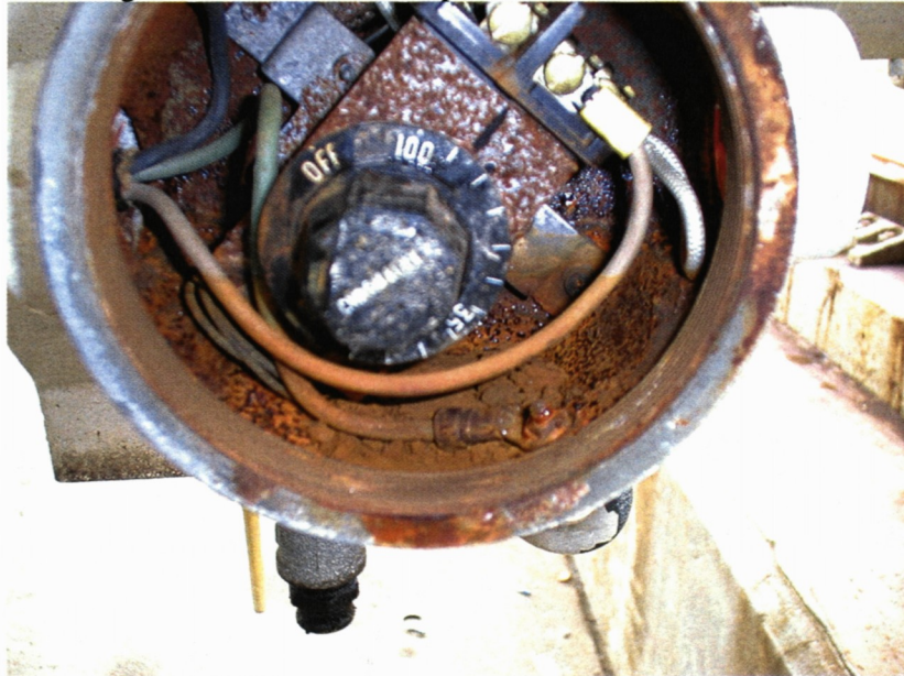
Figure 2: Gearbox Heater
