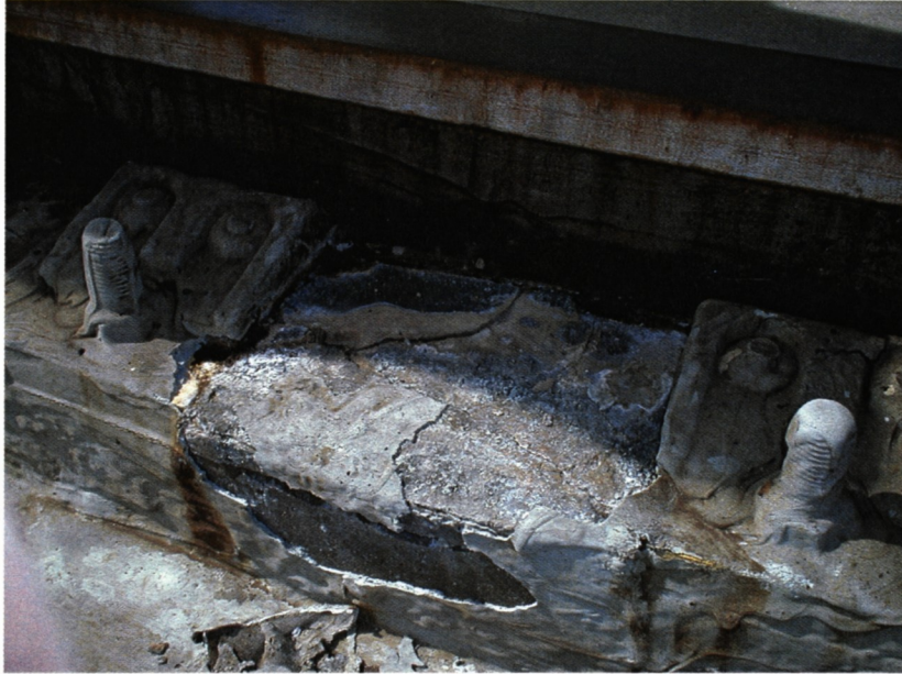
Figure 4: Grout Failure
