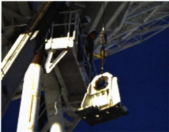
Figure 5: Pillowblock on the way down
