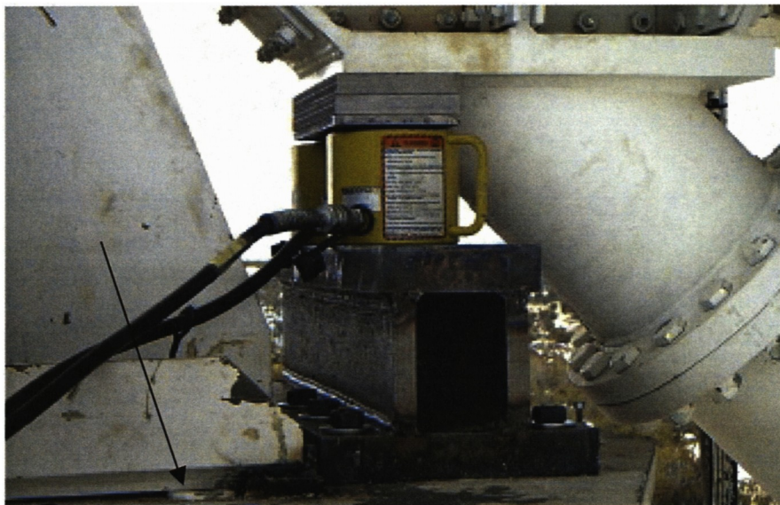
Figure 12: Detail of jacks. Note washers RSi used for shims under pillowblock.
