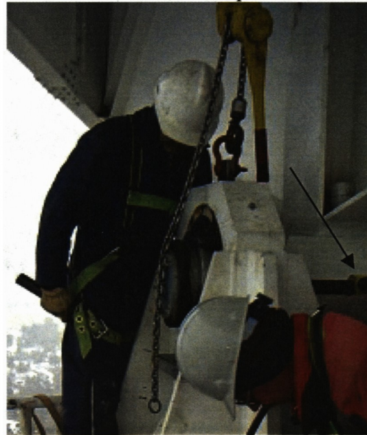
Figure 11: Small Porta-Power for removing PB
