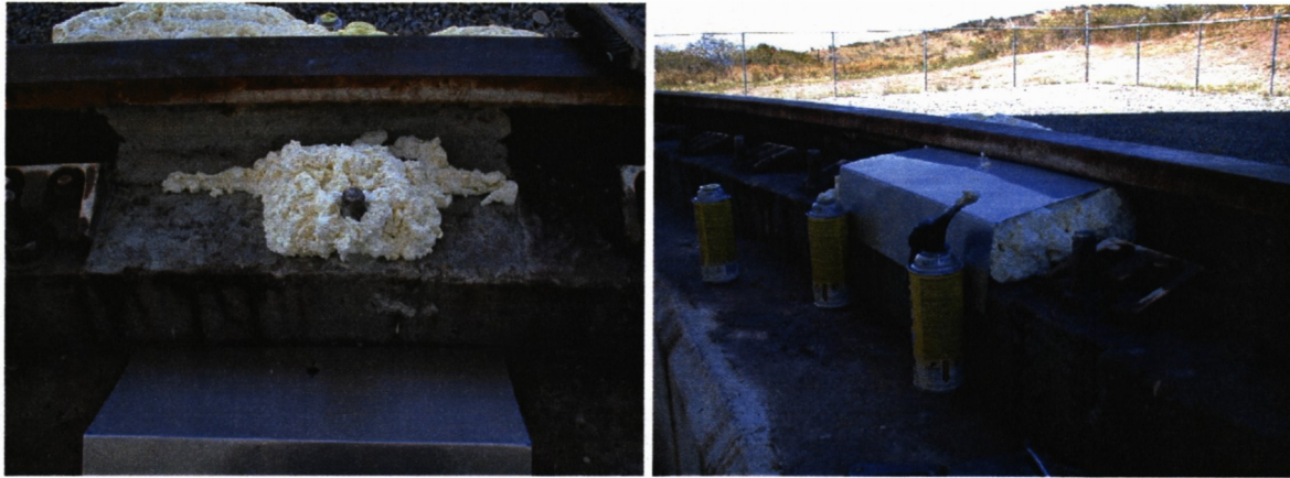
If we decide to foam the rails, aluminum flashing should be placed over the foam.
