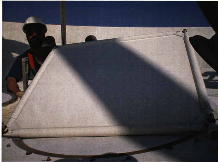
The dichroic panel is in good condition.
