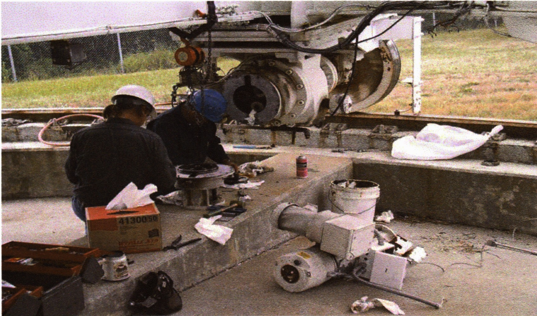
Azimuth #2 gearbox, 1 st and 2 nd stage gear inspection.
