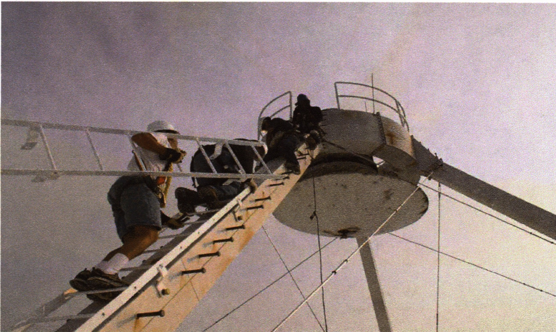
A new ladder and fall arrest was installed. Techs were trained on using the new fall arrest. Quad legs have a lot of surface rust.
