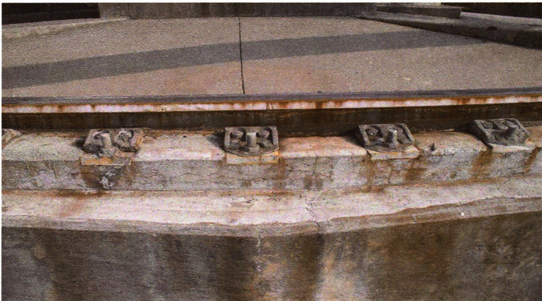
Rail is in good condition. Vulchem is deteriorating off all of the rail clips.
