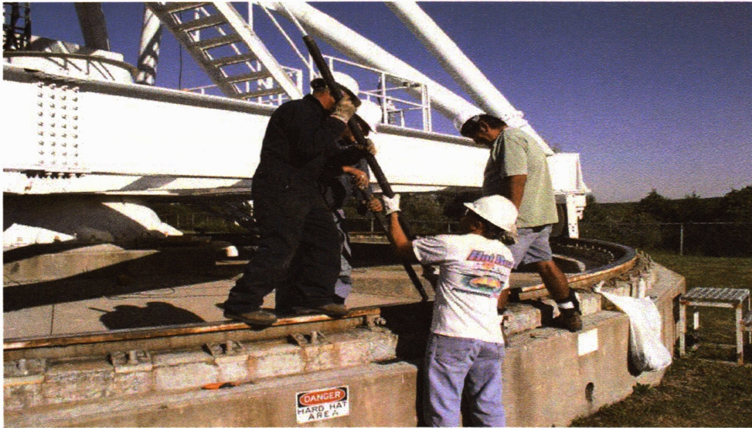
The guy's tightening loose rail splices. All splices were loose.
