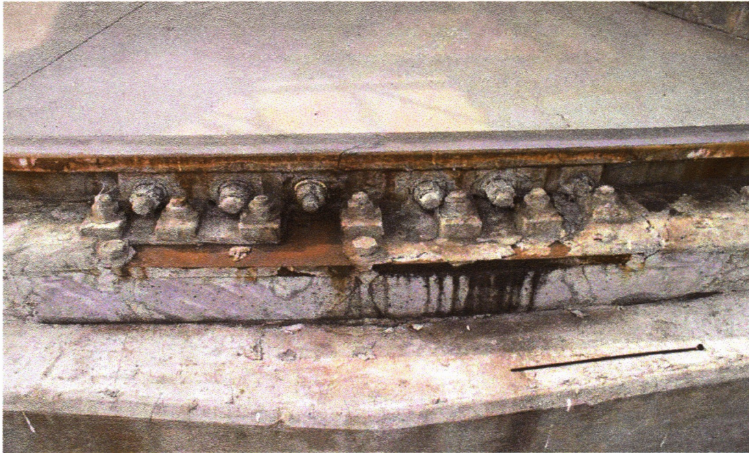
Vulchem is rapidly deteriorating from this rail splice and all the others.
