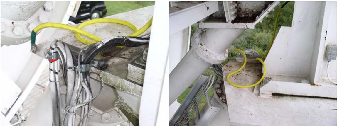
The synchro side elevation cable wrap was repaired by repositioning and replacing strain relief brackets. Both elevation ground cables were replaced.
