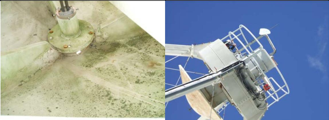
The snow tarp was removed and three 1 inch drain holes were drilled in the center of the sub reflector for drainage. The sub reflector was rebalanced. The rotation single motor modification was also completed.
