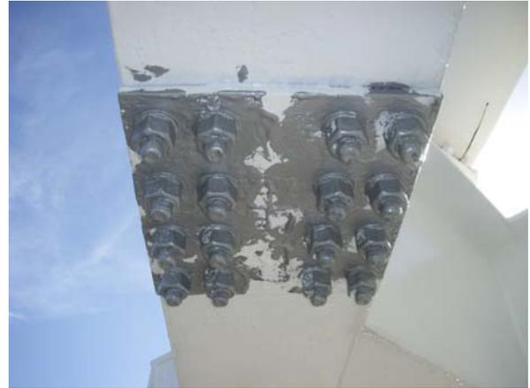
Some of the rust stained bolt heads and nuts were also painted by brush to inhibit further corrosion. Additional stripe painting of bolt heads and nuts should be performed in the near future to deter further corrosion.
