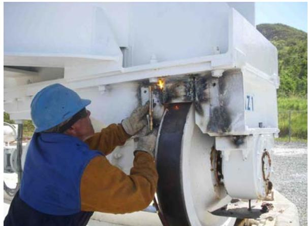
Both azimuth wheel assemblies were replaced during the maintenance period. Azimuth drive # 1 was an old style wheel/axle assembly that was replaced as a preventative maintenance measure. Azimuth drive #2 was a new style wheel/axle assembly that had metal particles in the grease on the inside bearing. This assembly was installed in 2000. This wheel/axle assembly will be disassembled and inspected to establish the cause of the bearing failure.
