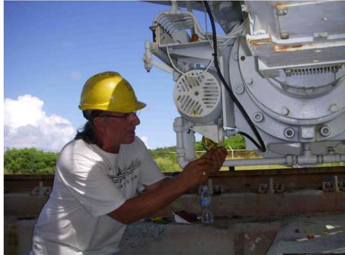
The insulation that was removed during the painting project was replaced. Traditional Tiger Team tasks and inspections were completed. These included: Focus Rotation Mount PM and Flex Shaft replacement, Azimuth and Elevation Gearbox inspections and oil changes, and other items as described in the Tiger Team task list. Numerous electrical repairs and inspections were made. These are listed in Appendix A.
