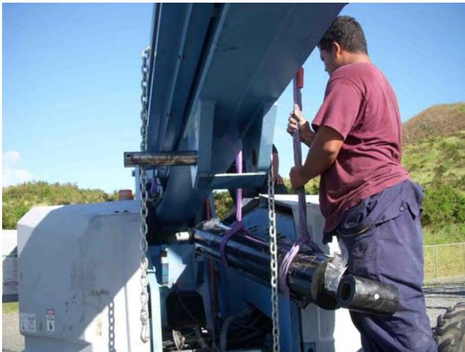
The boom lift cylinder, boom lift cylinder pins and basket cylinder pins were replaced on the Genie S-80 Manlift. These items were supplied by the manufacturer as part of a safety recall. This task was contracted to EM Solutions and was accomplished during the maintenance visit because the task required both a crane and a forklift. A crane and forklift were rented for this maintenance visit as they were needed to facilitate several of the tasks.
