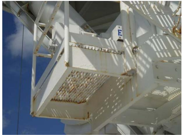
The elevation platform extensions and swinging platform have significant corrosion and will need to be replaced during a future maintenance visit. The hand rails on these parts of the structure are corroding from the inside out. A crane with at least 70 feet of stick will be needed to replace the swinging platform.
