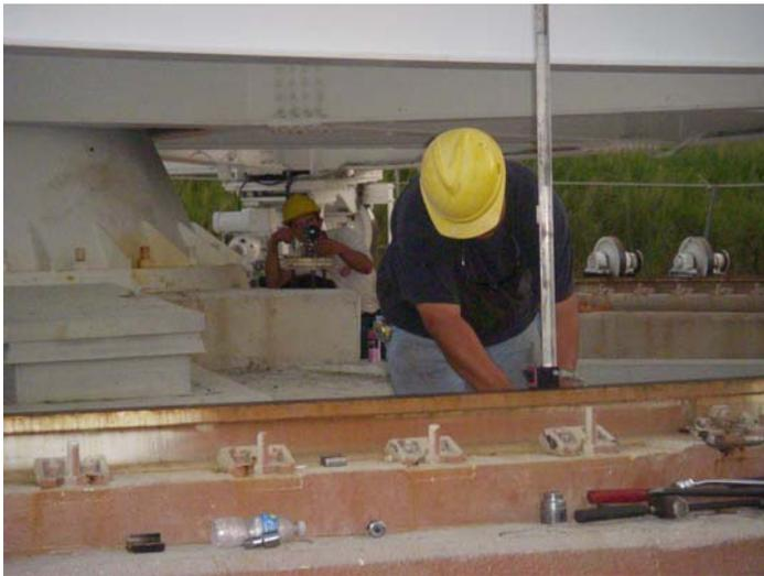
The azimuth rail was measured. As can be seen in the chart above, a low spot was developing at bolt number 119. This spot was repaired by installing shims between the rail and the splice plate. These shims should be monitored on subsequent maintenance visits to ensure that they do not initiate corrosion under the rail. A 0.080\"/>
