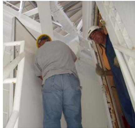
Other badly corroded items such as the step and door shown above were replaced. The new items had paint systems similar to the one on the HVAC platform described above. A finish coat of Acrylic Polysiloxane (Amercoat PSX 1001) was used on the door.
