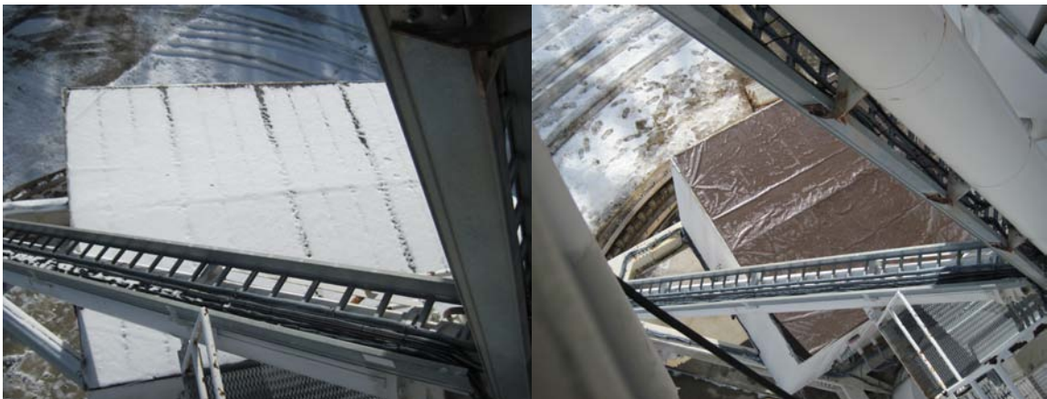
The antenna pedestal room roof has deteriorated so much that the site technicians attached a tarp to keep moisture from leaking into the Servo and FRM electronics. This roof needs replaced ASAP.
