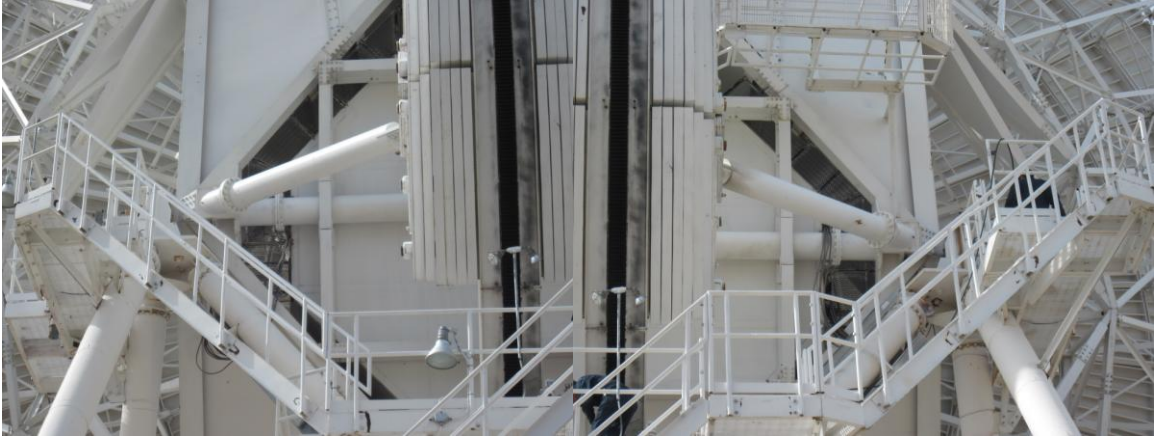
Elevation axle has no visible signs of cracks. Paint is in good condition.
