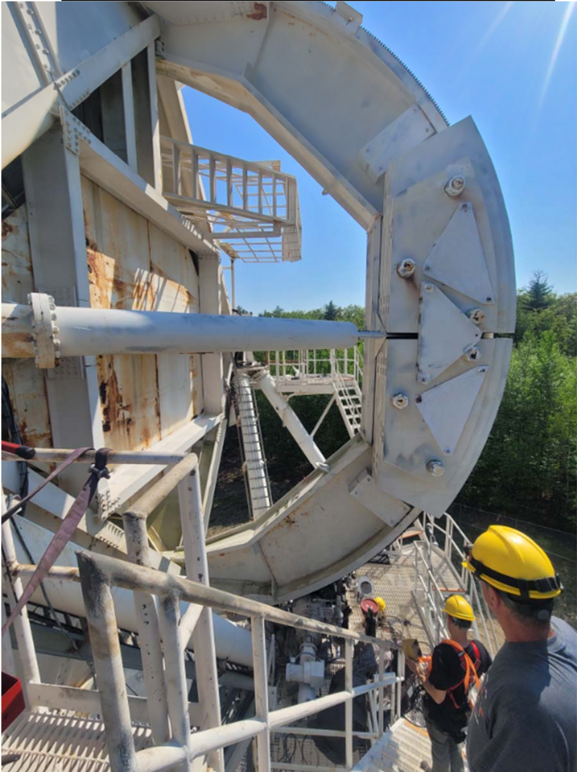
Figure 13: The dish was rocked back and forth repeatedly to ensure it was not making unusual sounds or movements.
