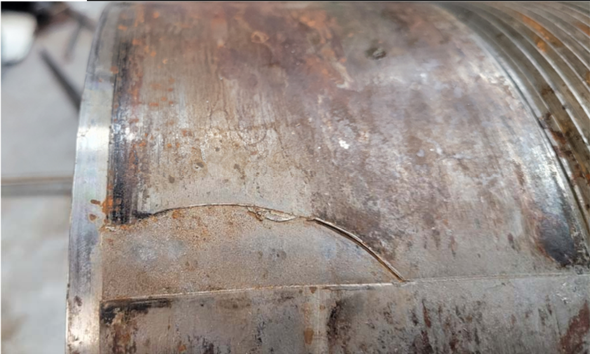
Figure 21: The marks on the taper coupling match up with the axial cracks on the inner race.
