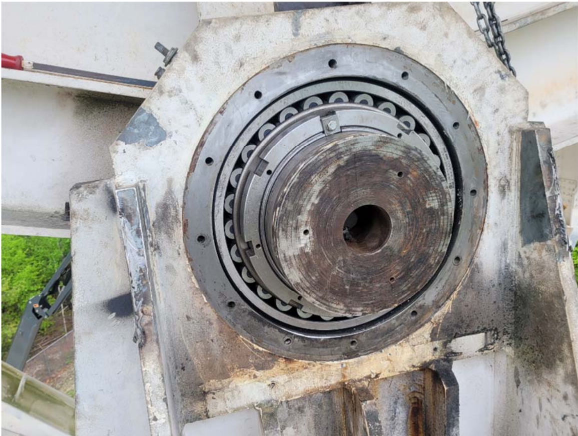
Figure 12: A newly installed bearing on the synchro side (before it had been greased.)
