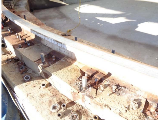
Figure 3.2.1: Rail with Clips Removed.
