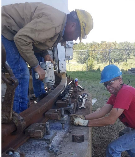
Figure 3.5.1: Rail Being Placed
