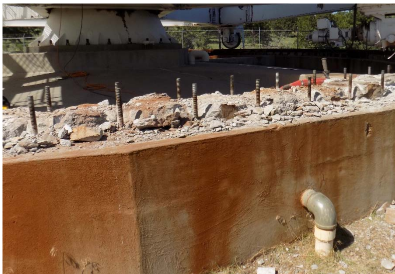
Figure 3.2.2: Old Grout Removed.
