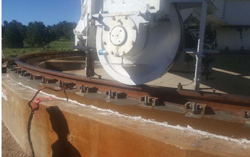
Figure 3.9.1: New Epoxy Grout Rail Bed.
