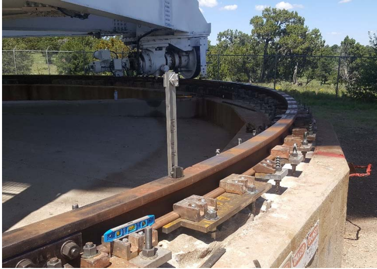
Figure 3.6.1: Level Target on Placed Rail
