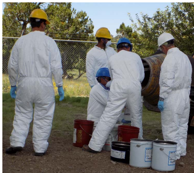
Figure 3.8.1: Mixing of Grout
