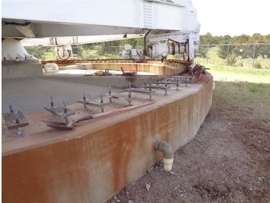
Figure 3.2.3: Rail Plates w/ Grout Removed
