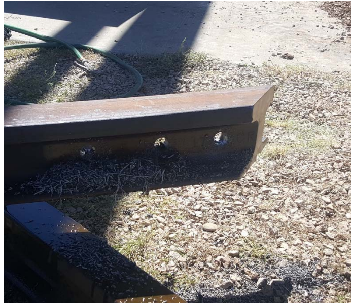
Figure 3.4.3: Splice Plate Holes
