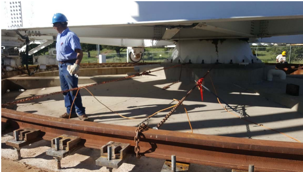
Figure 3.5.2: Rail Alignment using Chains and Binders
