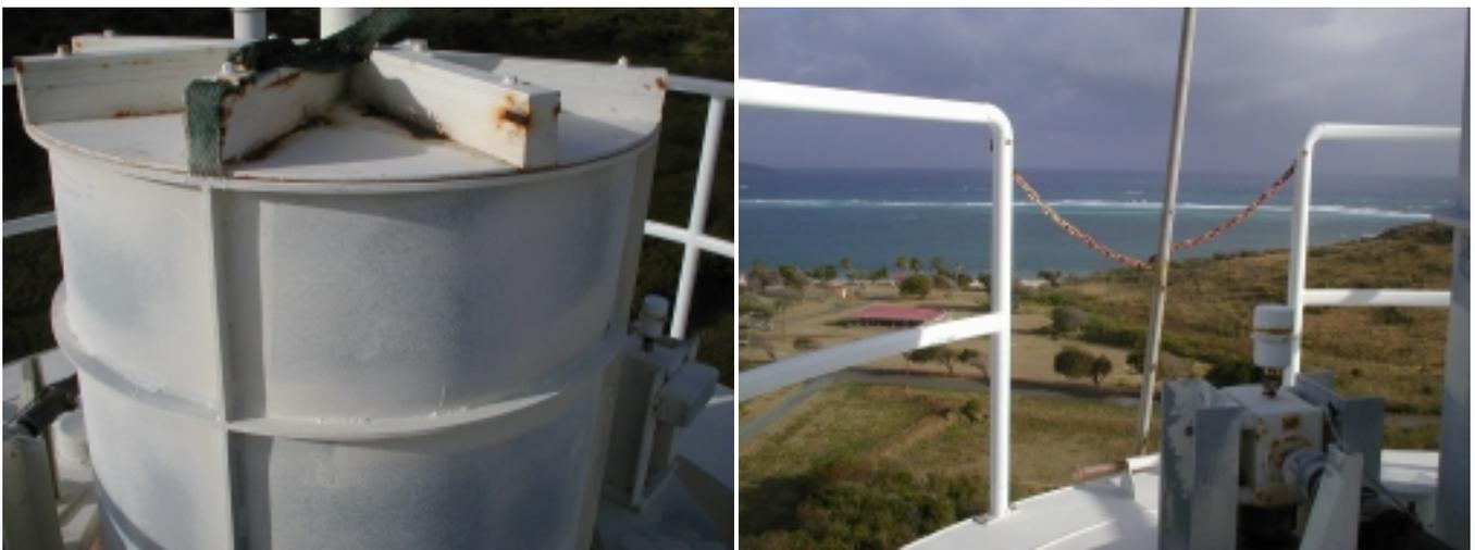
Some of the SR counterweight screws and the handrail chain were replaced.
