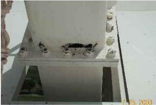
This picture shows a hole that has corroded all the way through the quad leg of the antenna. The steel on this side of the quad leg has completely failed due to this corrosion. The reason that the corrosion is so bad on this part of the quad leg is that water runs down the inside of the quad leg and pools on an internal lip in the quad leg. This quad leg should be repaired during the next maintenance visit.
