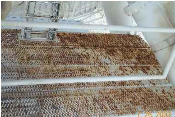
The walkway grating under the elevation platform has corroded to the point where it needs to be replaced during the next maintenance visit. The metal has corroded away so much that I was able to easily knock holes in the grating with a small hammer. The cable tray should also be replaced during the maintenance trip.
