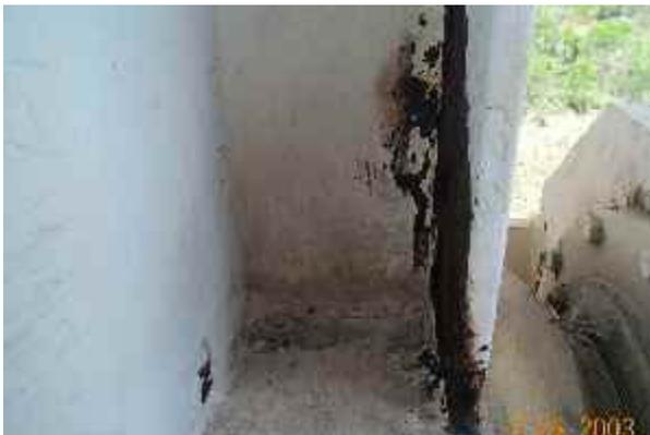
The major structural elements of the antenna were not severely corroded except for one of the beams that connect the dish to the elevation axle. Approximately 20% of the flange thickness has corroded away. This beam is in a pocket on the up side of the antenna where water collects. It will be very hard to drill a drain hole in this pocket. Therefore, the site techs should “Chem Prime” and paint these areas carefully.
