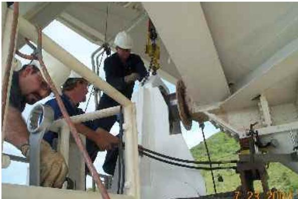
It was not possible to gain access to a large press on the island of St. Croix, so instead of risking the possibility of not being able to remove the old bearing from the bearing pillow block, a new elevation pillow block was fabricated and installed with the new bearing.
