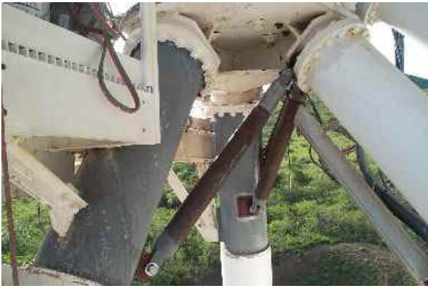
During the Las Alamos elevation bearing change, we experienced deflections in the antenna structure that were greater than were desired. Therefore, the finite element model was refined to better simulate the entire structure under the load path required for the bearing change. Using this model, it was found that installing the two struts shown in the photo in addition to the jack support beam, brace beam and anti-rotation pin that were installed in Las Alamos as described in
