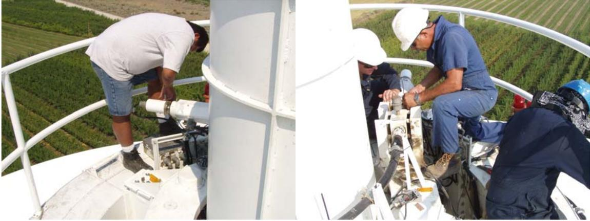
FRM was given a thorough inspection. A focus flex shaft was replaced and the new encoder coupling modification was installed.
