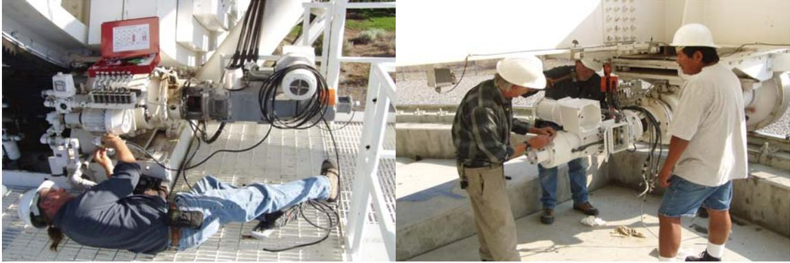
New digital tachs were installed on EL and AZ motors. All AZ and EL lube pump SJO power cables were replaced. Azimuth #2 motor was replaced. The ACU power supply and backplane upgrade were installed and tested.
