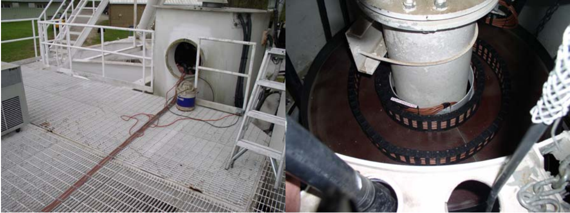
The new IF Cable Wrap was installed and tested.
