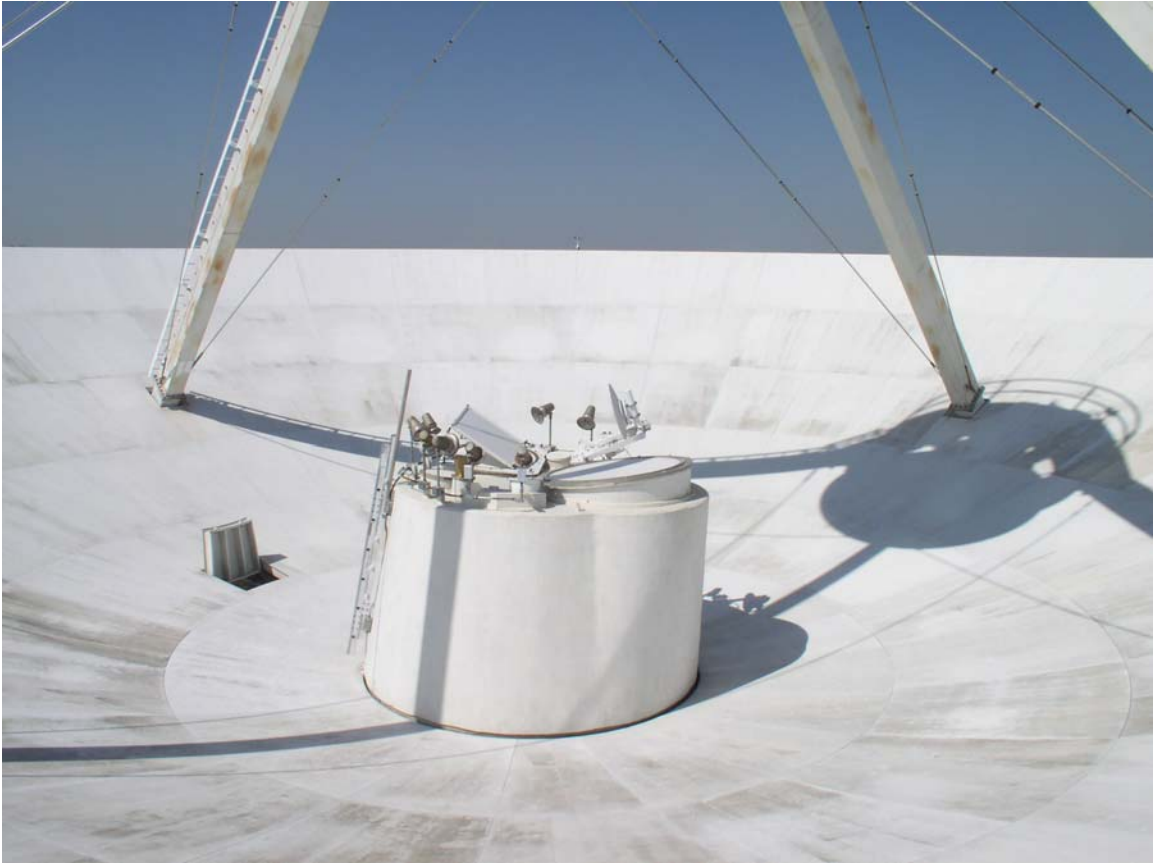
Dish panels are in good condition. The feed cone's elastomeric paint is holding up well. The feed cone was sealed and painted back in 9/2003.
