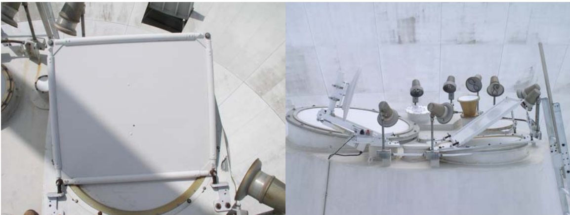
Dichroic reflector is in good condition. Ellipsoid reflector is in good condition. Dichroic reflector actuator operates correctly.
