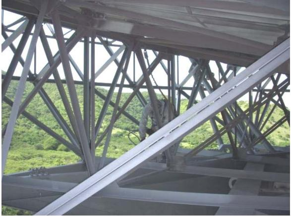
Figure 8, Backup Structure Truss Epoxy Intermediate Coat.
