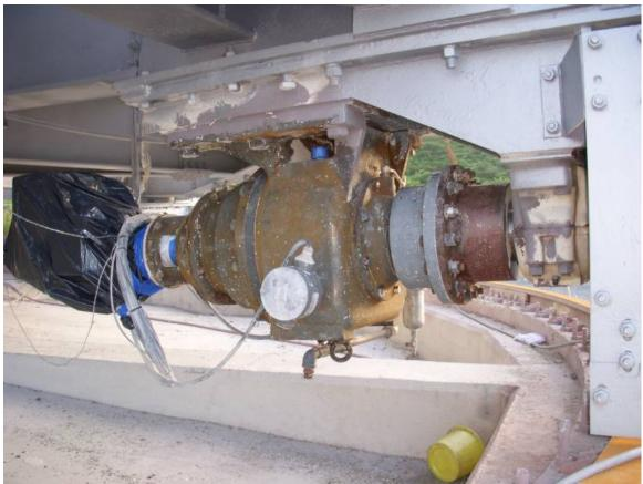
Figure 5, Power Tool Surface Prep on Azimuth Drive Gearbox.
