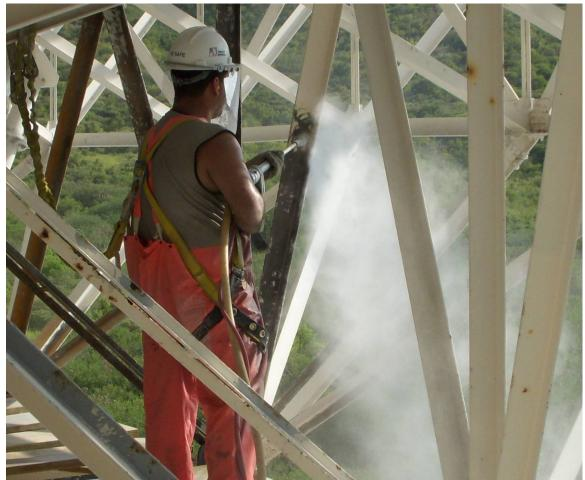
Figure 2, Ultra High Pressure (UHP) Waterjetting Structure at 42,000 PSI
