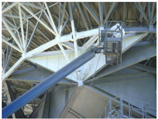
Figure 1, Applying Topcoat on Structure
