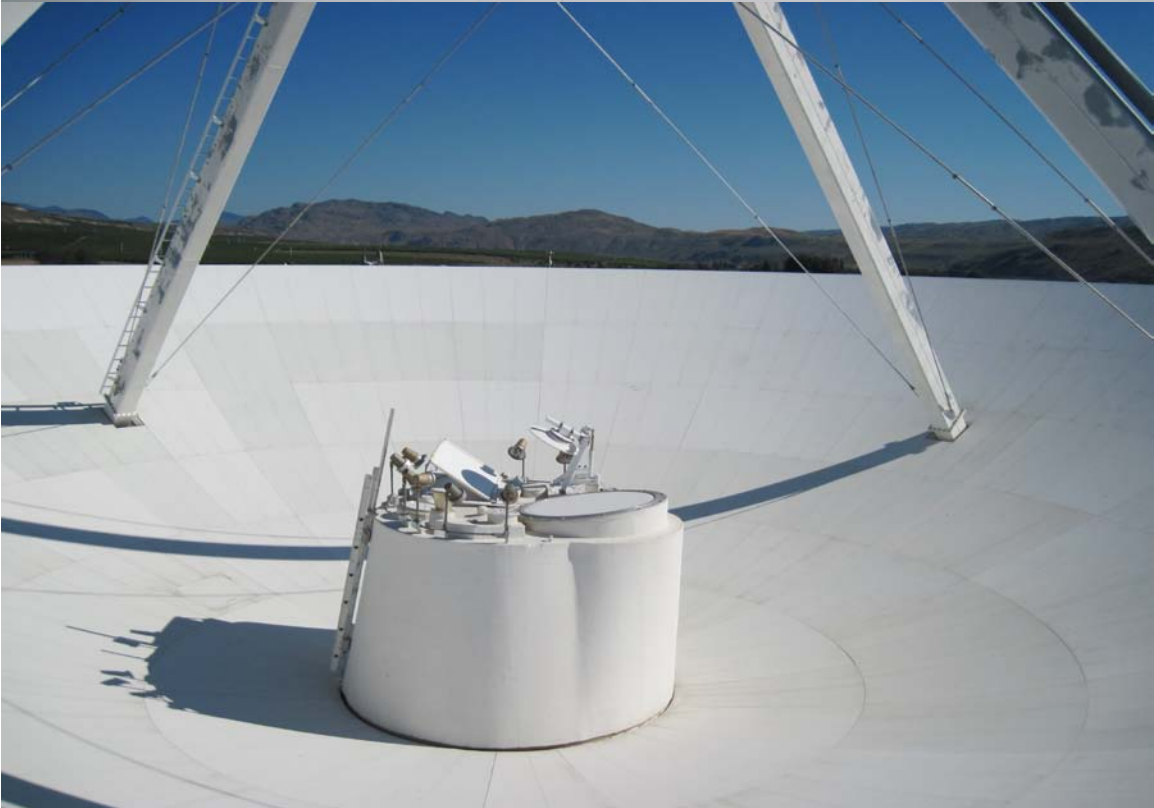
Dish panels are in good condition. The feed cone's elastomeric paint job is holding up well.
