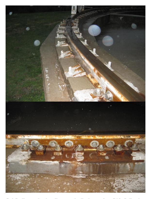
Bob Broilo completed a rail grout and splice bar repair on 7/10. Rail and grout is in great condition. Page 7
