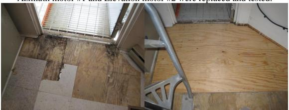
The Vertex room floor was severely rotted and had to be replaced.
