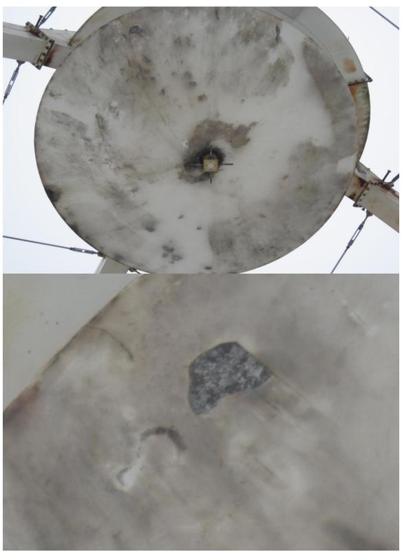
Sub reflector paint is beginning to flake off. FRM was given a thorough inspection. The focus flex was replaced. The FRM is well lubricated.
