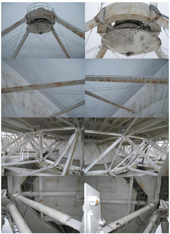
The Antenna needs some "spot painting" or a complete paint job. Paint is flaking off and surface rust is affecting most areas of the Antenna structure.
