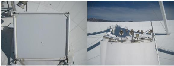
Dichroic reflector is in good condition. Ellipsoid reflector is in great condition and the actuator operates correctly.
