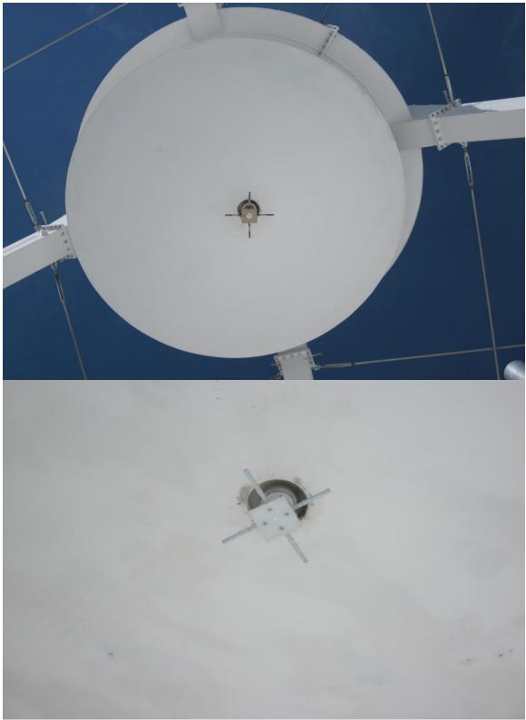
Sub reflector paint is in great condition. FRM was given a thorough inspection and the focus flex shaft was replaced. FRM is well lubricated. Page 2
