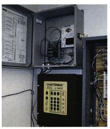
Remove the existing relay in the number 4 spot (on top) and install the Opto 22 ODC5R reed relay. Bring the wire up to the relay box and connect the other end of the wire to terminals 8 and 9 on the output strip (Relay 4 output connections).
