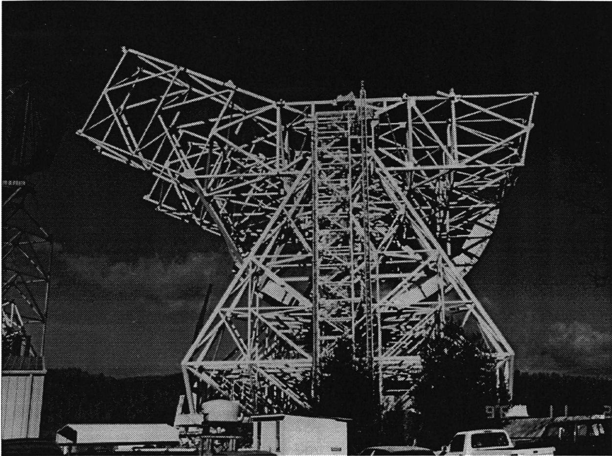
The GBT continues to grow at a steady pace. This picture, taken in December 1996, shows the horizontal part of the feed arm extending to the left. In January, this has extended further, and soon the vertical part will begin to be assembled.
