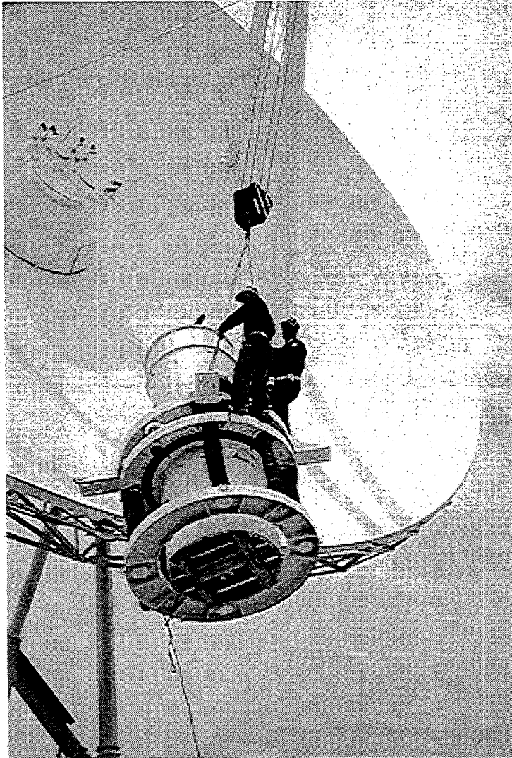
Figure 1, Left: John Wall and Malcolm Peralta ride the focus/rotation mount to the antenna apex at Los Alamos, June 1989.
