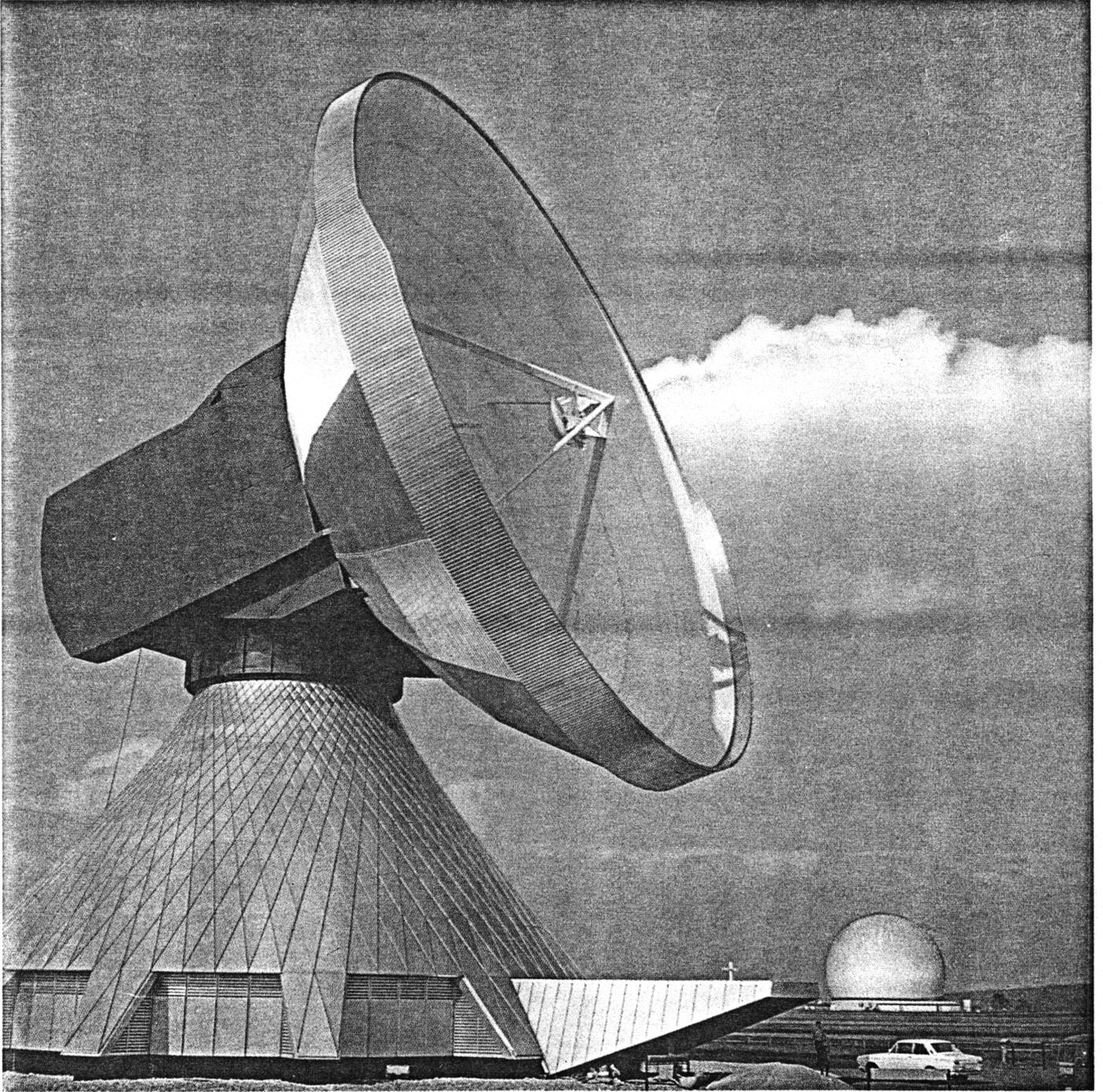
FIG. 2. Communication Antenna No. 2 in Raisting, Germany, has an insulation envelope similar to that proposed for the 30-m radio telescope.
