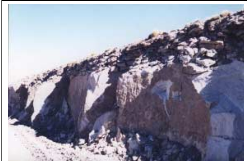
Figure 7: Cut along Jama road (A. Otárola)
