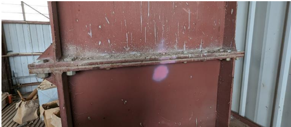
Figure 1: Typical column bolting section (12b)
