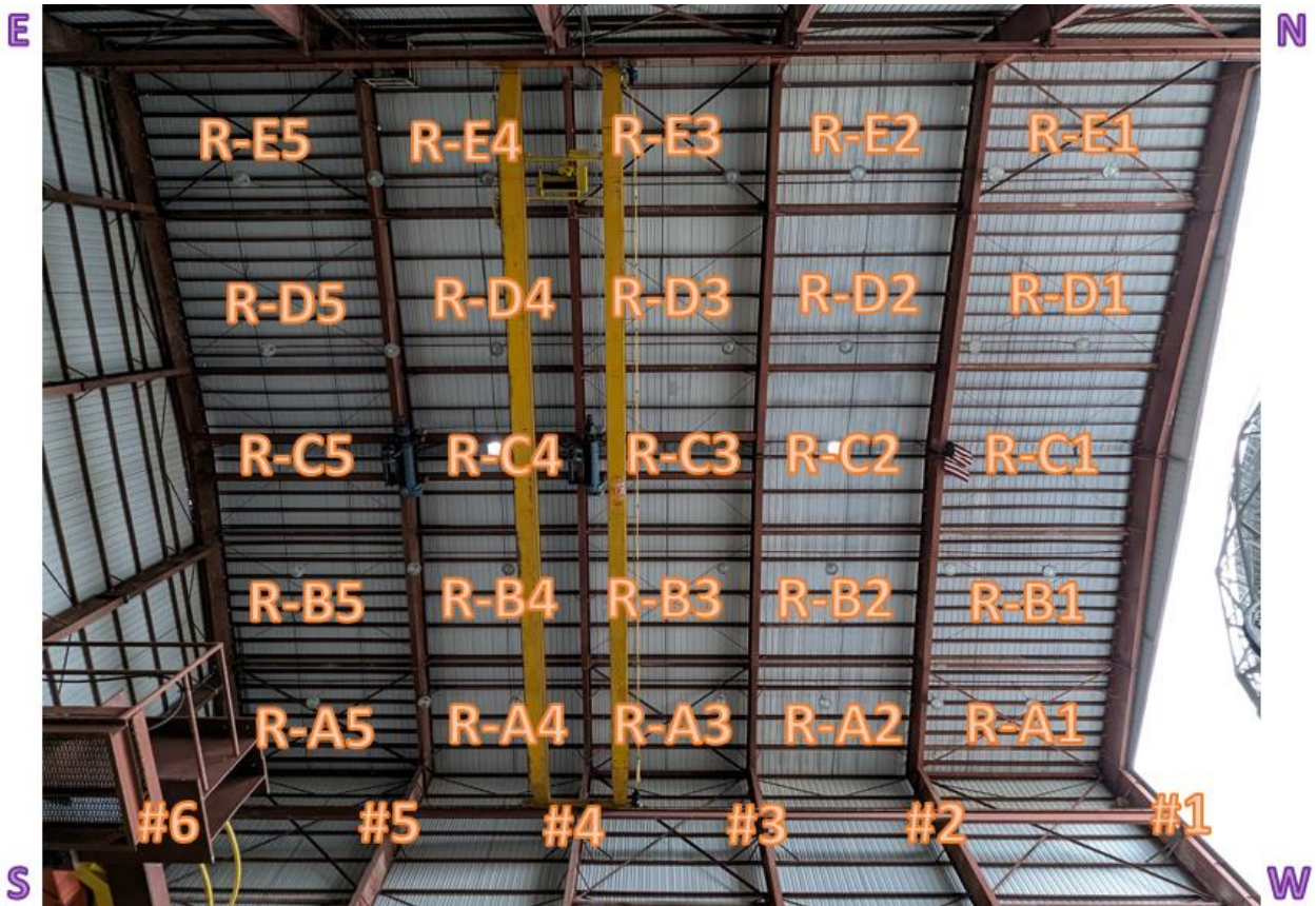
Figure A5: Roof labeling system.
