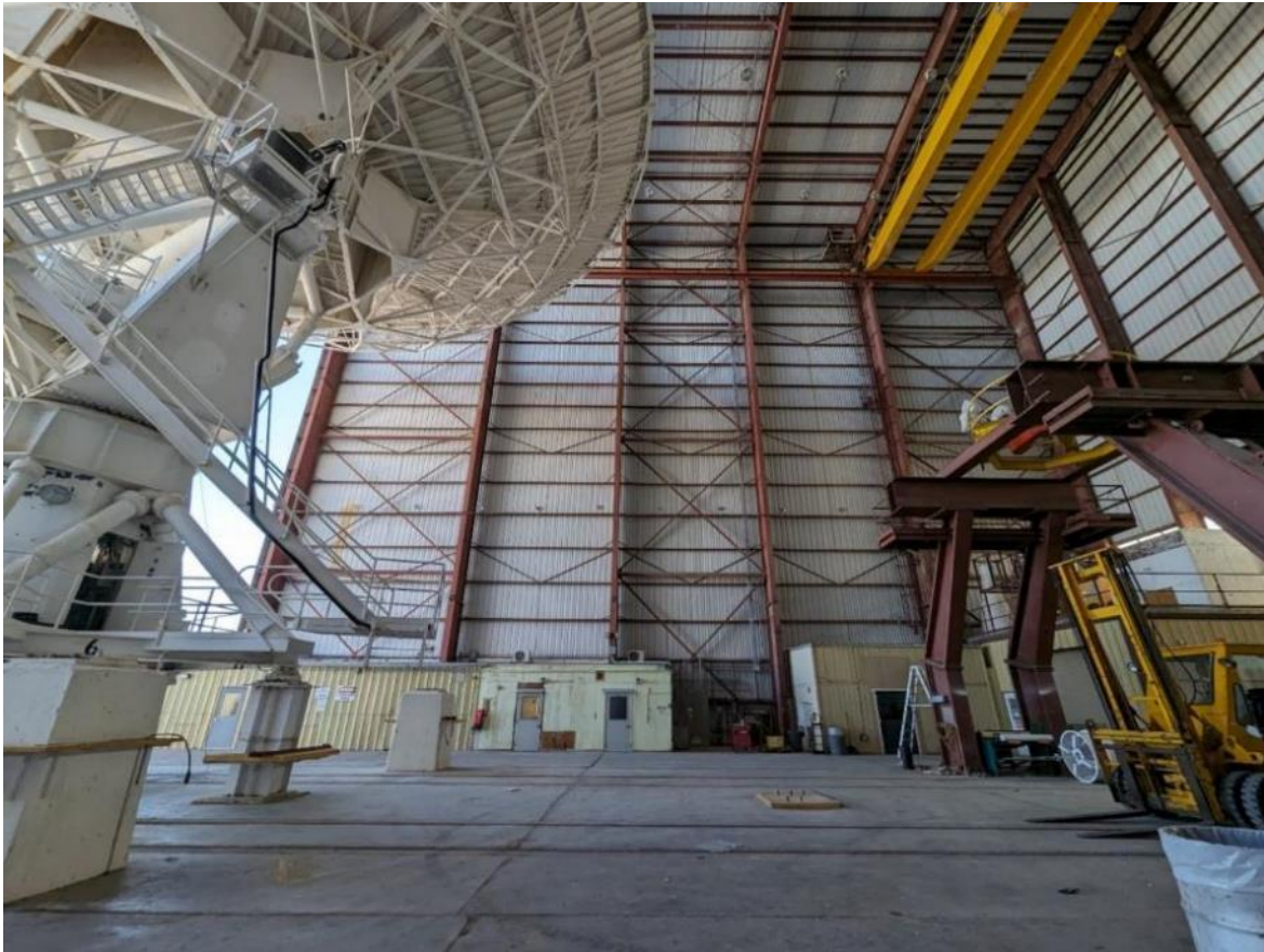
Figure 2: Inside view of Antenna Barn facing east wall with 6 columns.
