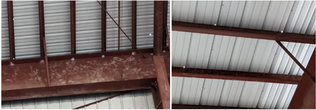
Figure 33: Left – 3 small visible holes (8d bottom right of image). Right – 3 more holes (R-B5, between 5e & 5f).
