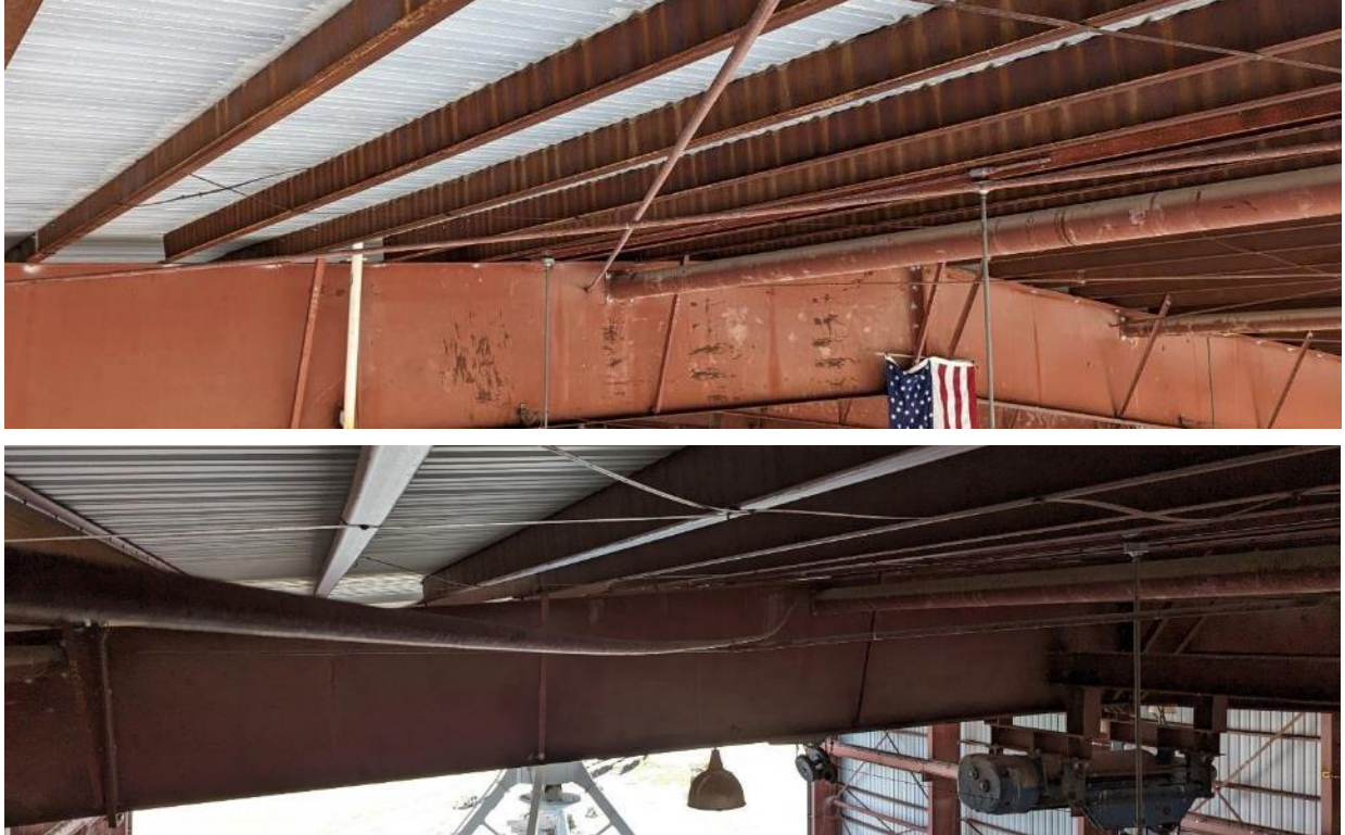
Figure 24: Top – Better tensioned cross rods (R-B1). Bottom – Members loose and fallen (R-B5).
