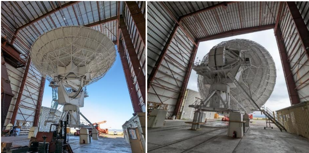
Figure 5: Left – Antenna before tilting. Right – Antenna after tilting.
