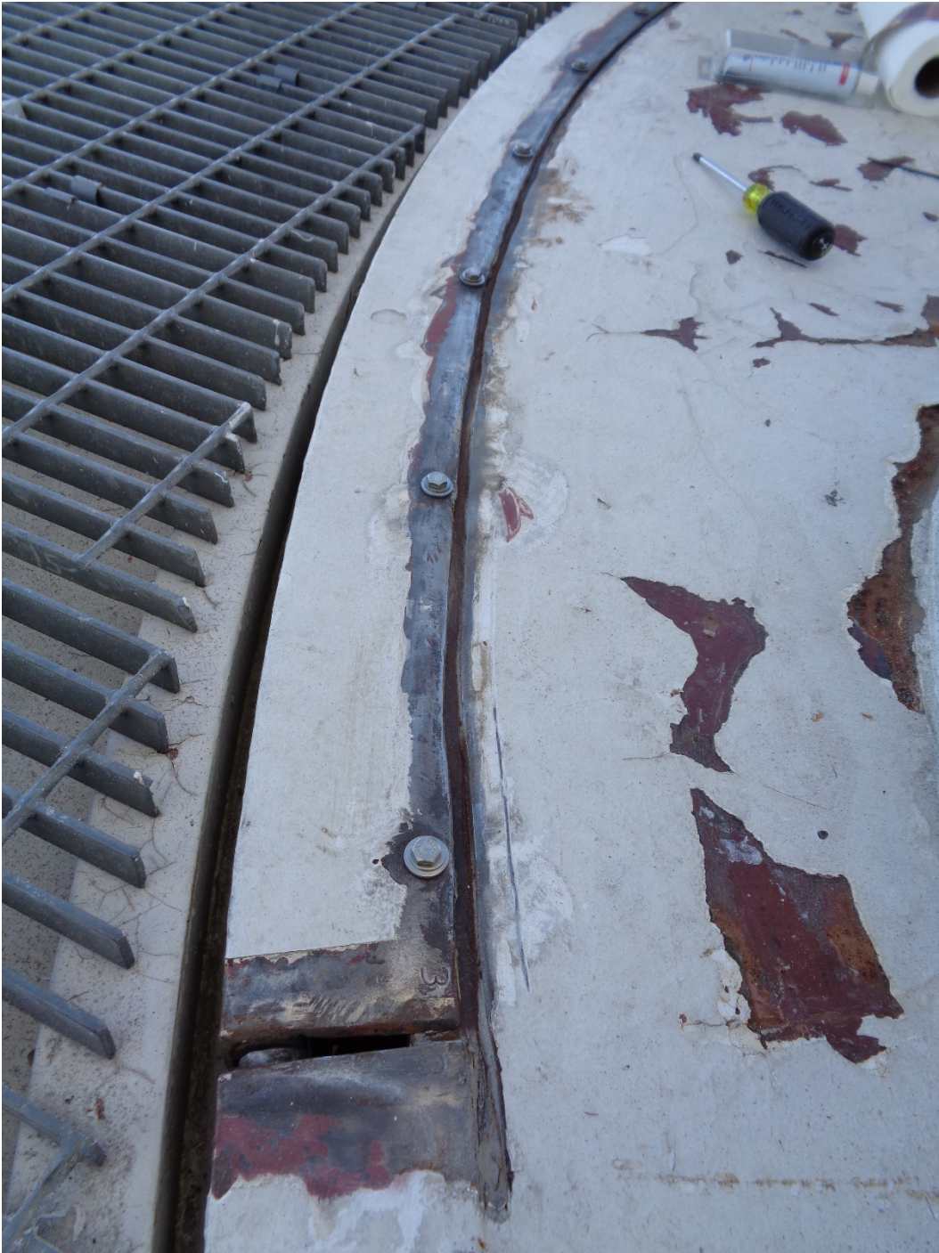
Cleaned rail section reinstalled with new hardware:
