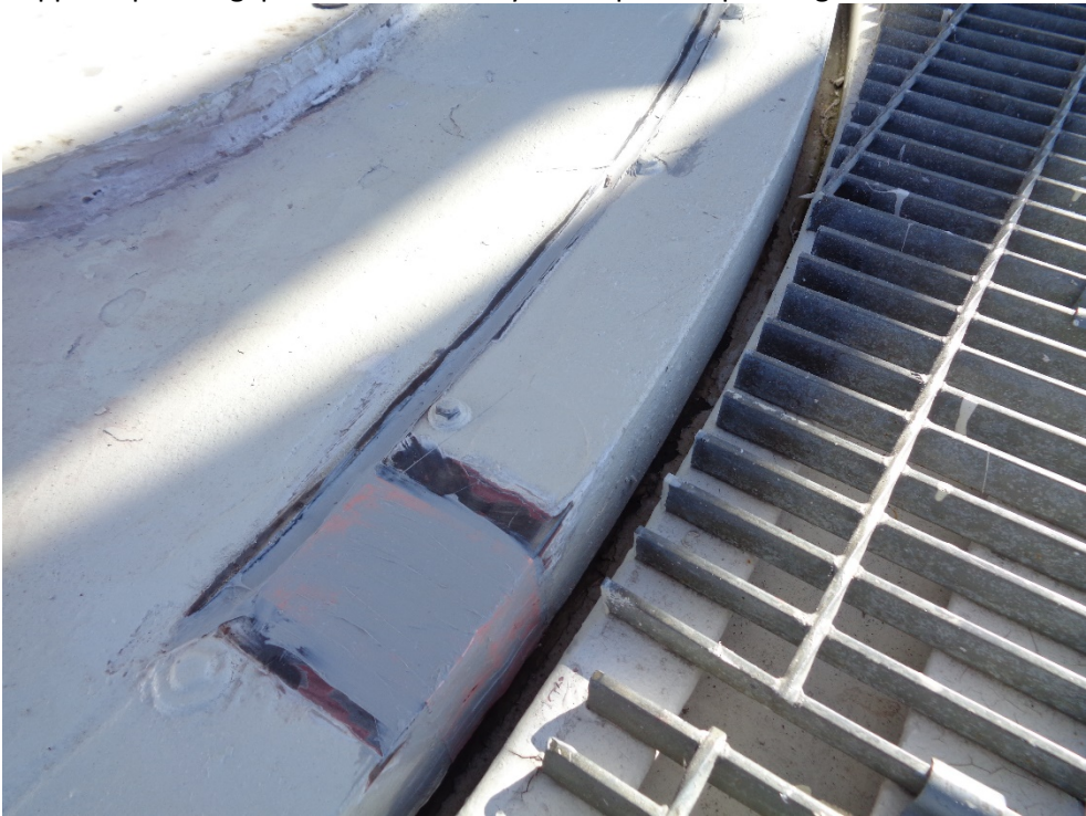
Copper tape and gap covered with Butyl caulk prior to painting:
