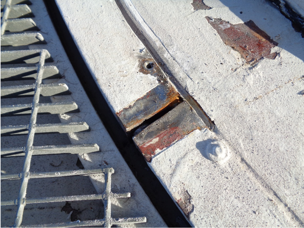
Old caulking, bolts, and copper tape between rail sections removed:
