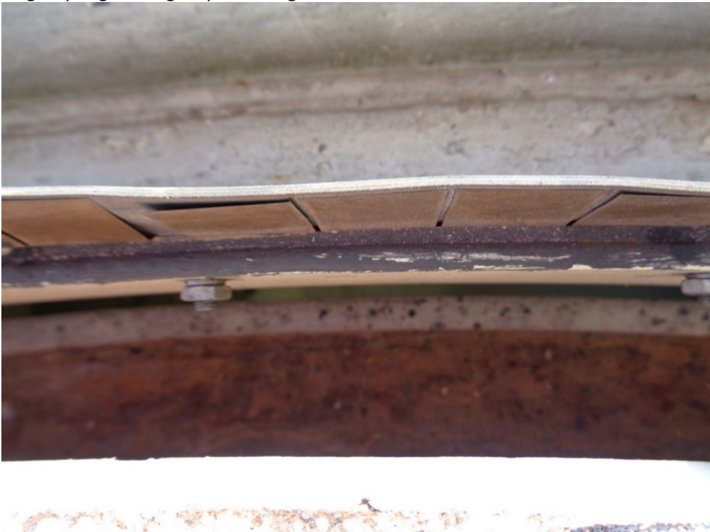
Finger spring backing strip and RFI gasket:
