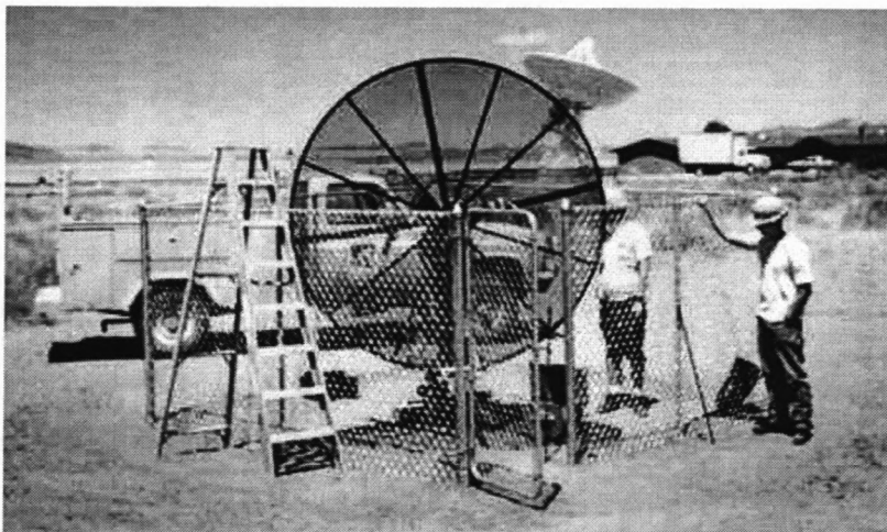
Figure 3.4.1 Reassembling the SRT at the VLA Site
