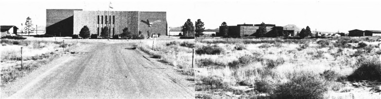
Figure 1-1. Photographs giving a panoramic view of the VLA buildings. The top picture, taken from the main entrance road, shows the bunkhouse trailer at the left, then the antenna assembly building, technical services building, and warehouse buildings. The center picture shows the sculpture in front of the control building, with the library/office building in the background. The bottom picture shows the control building, cafeteria, and visiting scientist quarters as viewed from the entrance road.
