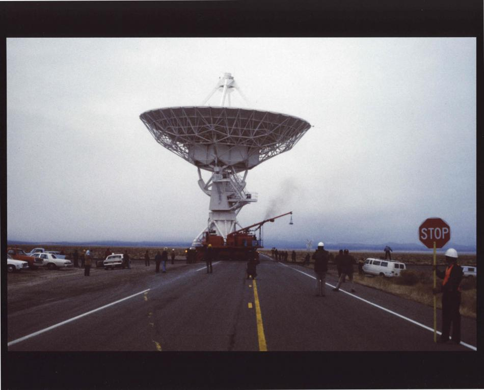
VLA Photo No. 4. A 100-foot high VLA antenna and transporter crossing U.S. Route 60 on its way to a foundation on the north arm of the "A" array. This was the first antenna to cross Route U.S. 60 and arroused much media attention.
