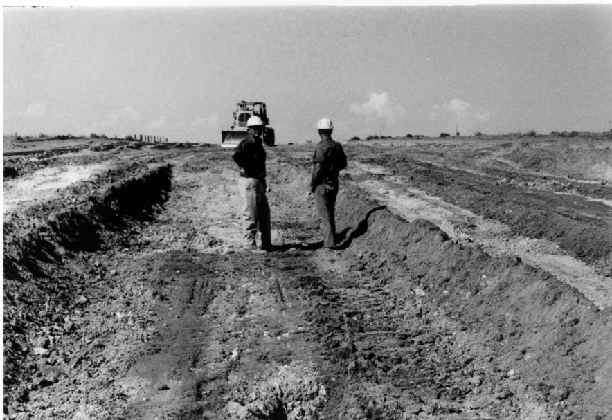
(p8-1) 8-14-74: VLA Site showing a view on the Southwest Arm of the Wye where a 2' - 0" layer of unsatisfactory earth had to be removed before construction of the railroad embankment could commence.
