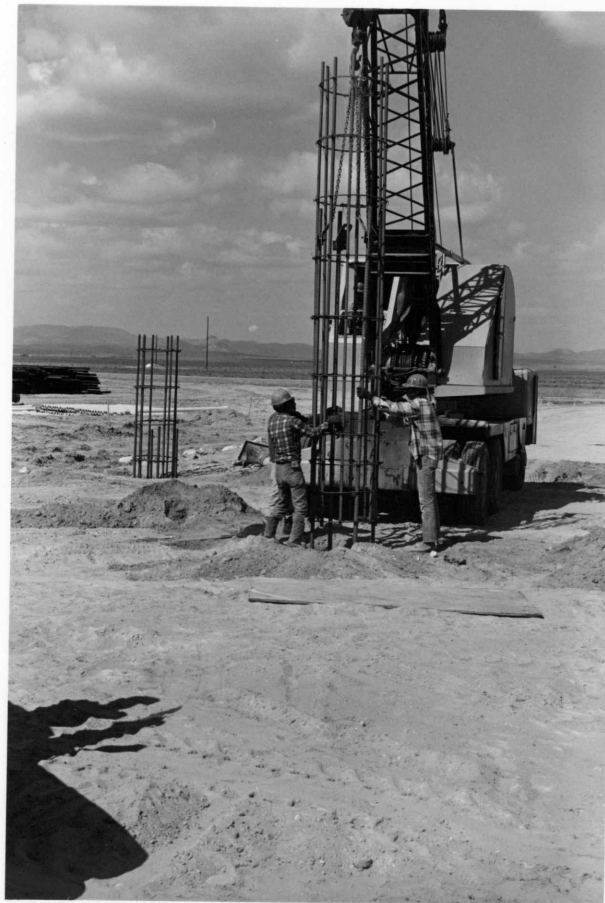
(p10-7) Emplacing the reinforcing steel for the piers in the antenna assembly building.
