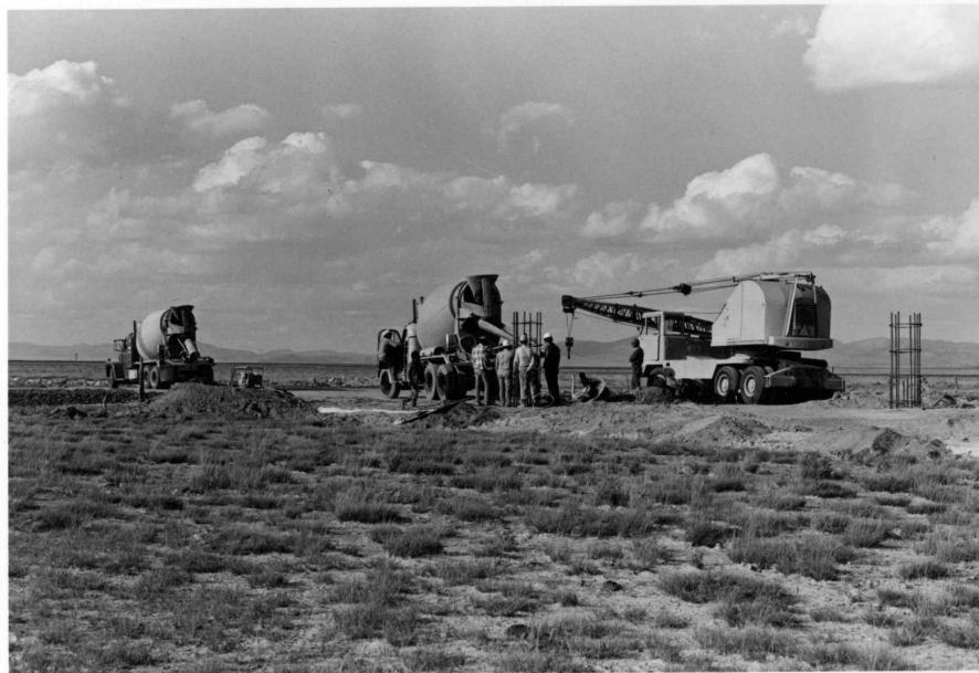
(p10-8) Pouring concrete for the piers of antenna station CW5.
