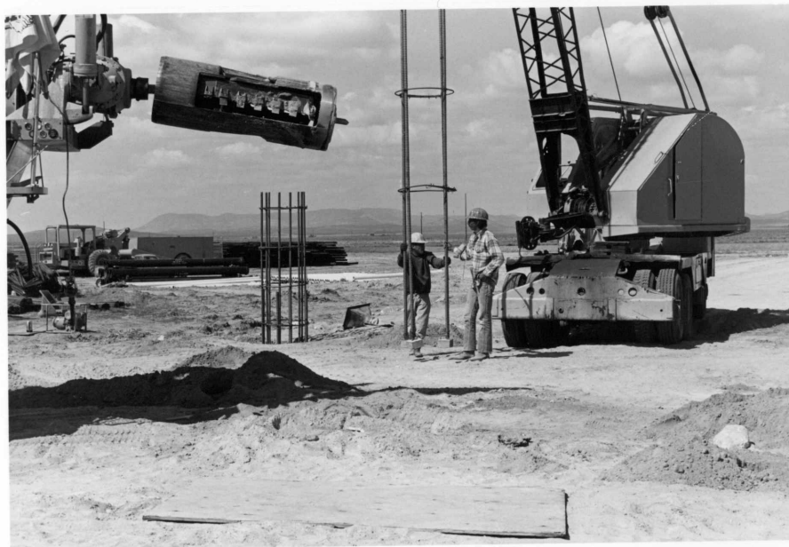
(p10-5) Emplacing the reinforcing steel for the piers in the antenna assembly building. Note rig used to bell the piers in the foreground.
