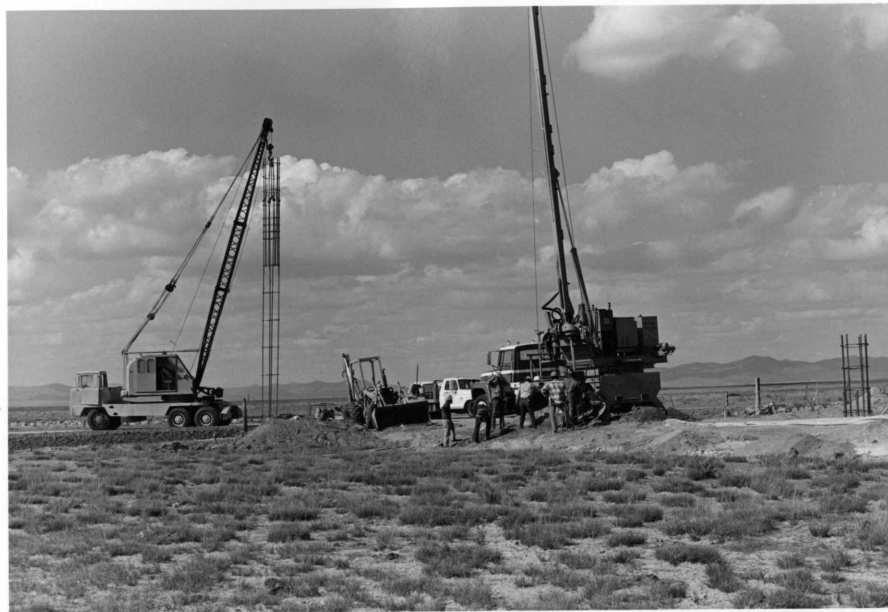
(p10-3) Drilling foundation piers for antenna station CW5. Note the pier reinforcing steel held by the crane.
