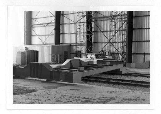
p2-75-1 Partially completed transporter frame inside of the Antenna Assembly Building.
