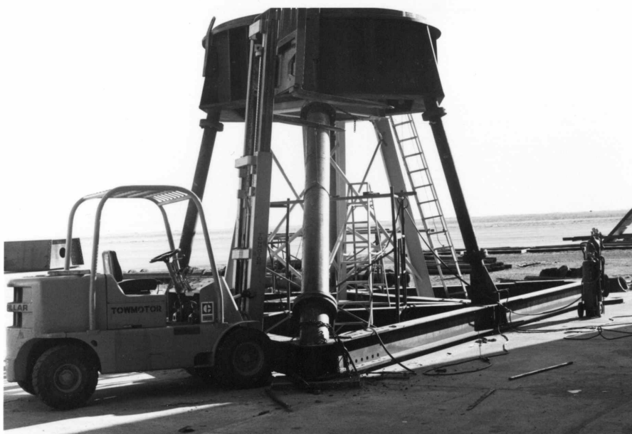
Antenna Pedestal with Bearing Support Mount at Hobbs, New Mexico
