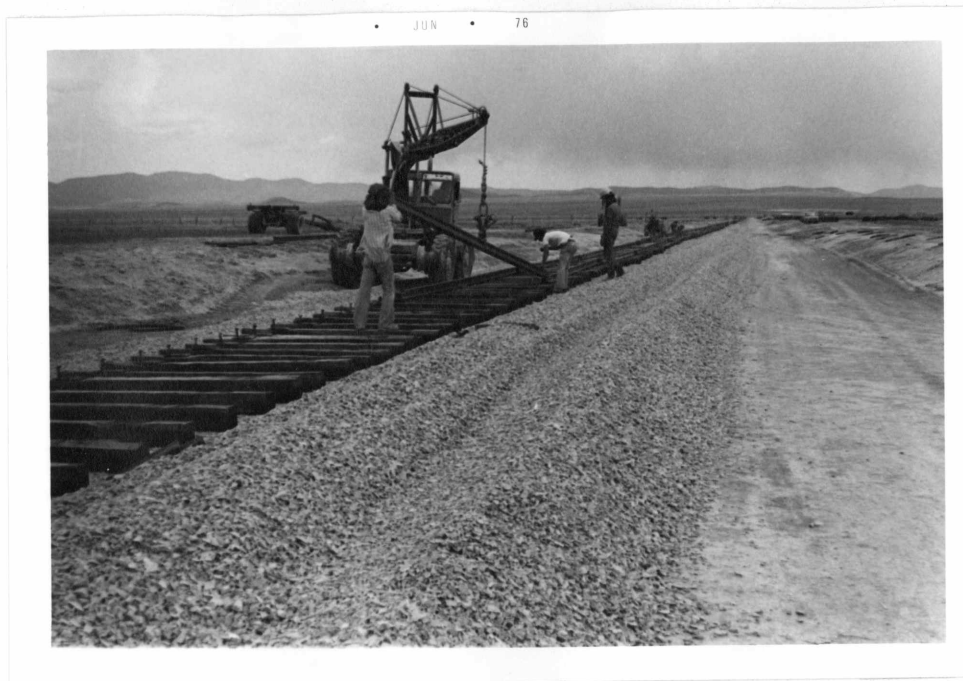
Assembly of Track at CN9
