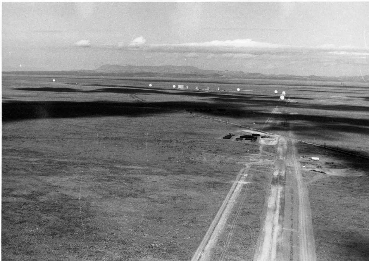
p10-78-1 (4A) Aerial View to Northwest of East Arm of Wye Showing Waveguide Excavation on left, Track Excavation and Grading on right. Rail and the Stockpile near Antenna Station BE7.
