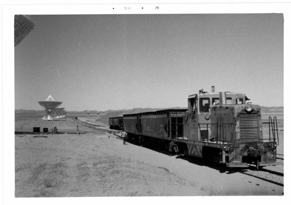
Diesel Engine Returning Cars to Load Ballast for East Arm Construction
