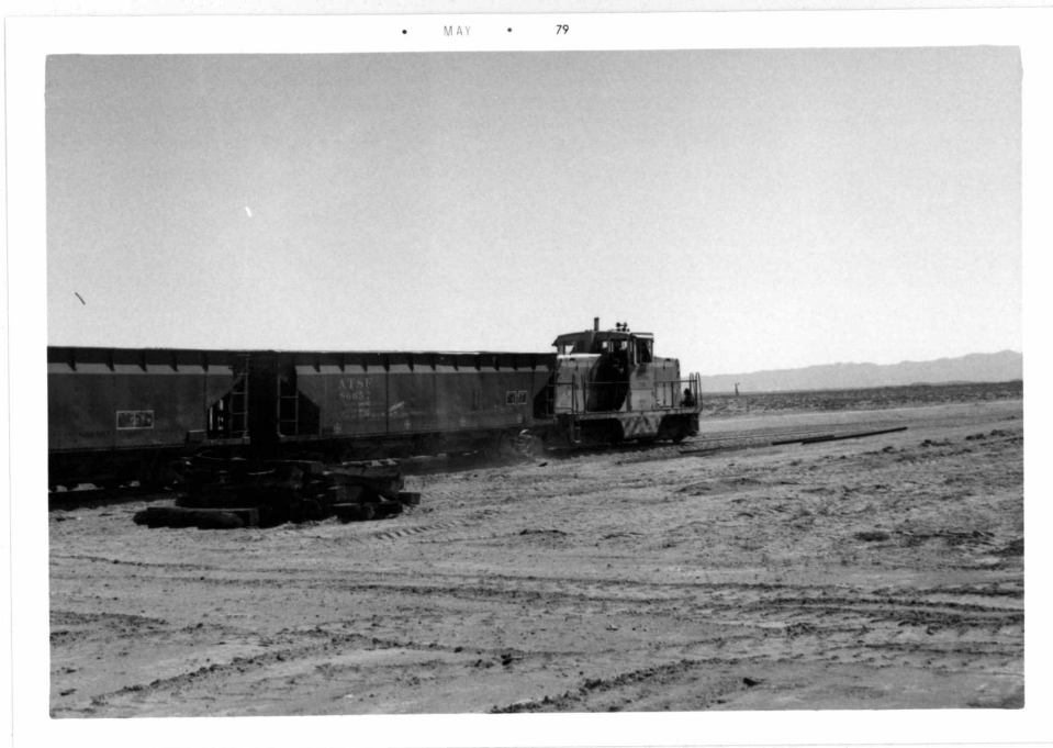
Pacific R.R. Construction Co. Diesel Engine Spreading Ballast on East Arm Construction
