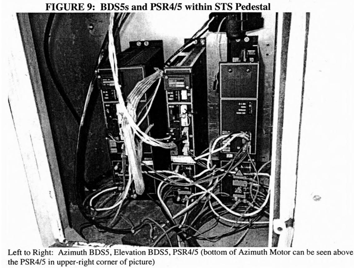
Left to Right: Azimuth BDS5, Elevation BDS5, PSR4/5 (bottom of Azimuth Motor can be seen above the PSR4/5 in upper-right corner of picture)
